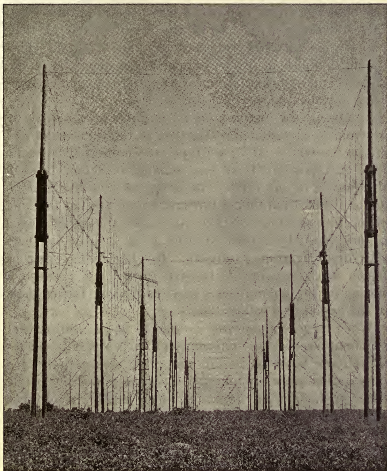
Beam antenna and line of towers for long-wave antenna, Rocky Point, Long Island, New York, station. (Courtesy of Radio Corporation of America.)
