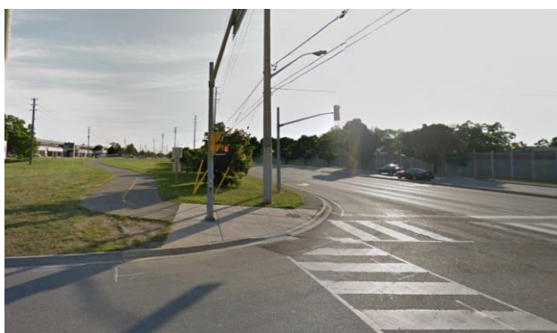
Multiuse path on The Queensway in Mississauga
