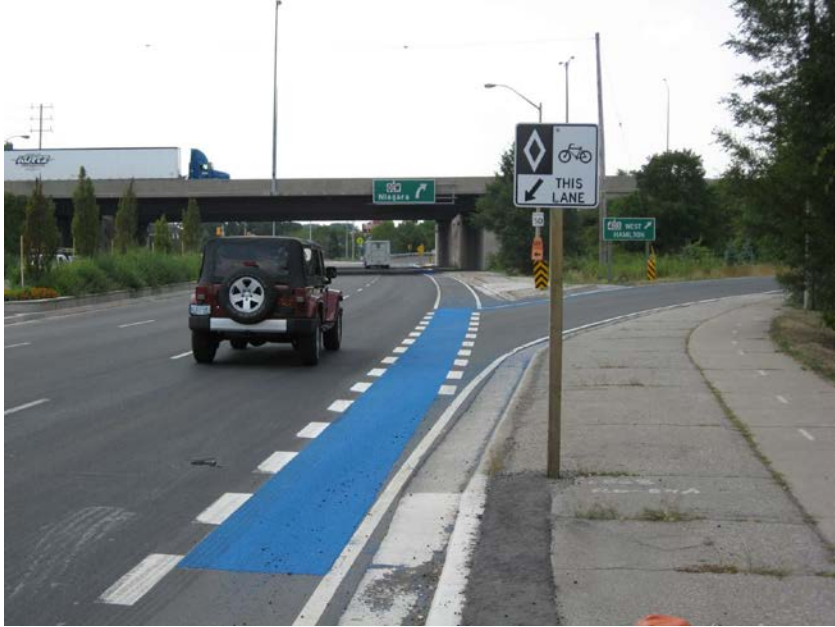
Figure 5- Completed Fairview Interchange
