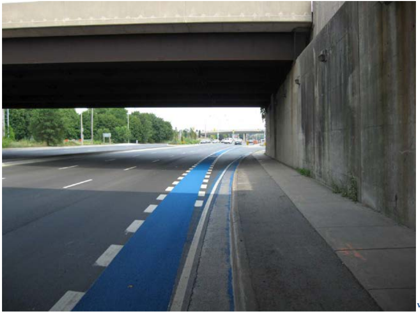
Figure 6 - Completed Fairview Interchange
