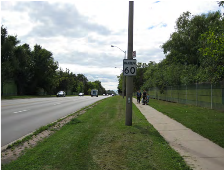
Figure 18: Finch Avenue West, looking west from Islington Avenue. High sound barriers line the road between Kipling and Islington Avenues, dividing the neighbourhood and increasing pedestrian travel distances.
