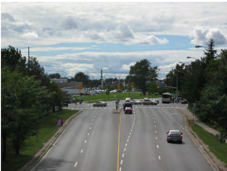
Figure 16: Finch Avenue West looking west towards Kipling Avenue. Wider road lanes with turning lanes at the intersections make the roadway more difficult to navigate for children, seniors and persons with disabilities by extending the distances they need to travel and exposing them to more lanes of traffic.
