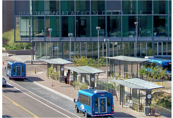
FIGURE 11. Dedicated pick up/drop off facilities for shuttle or ride-sharing services can help improve service and increase the attractiveness of these options.
