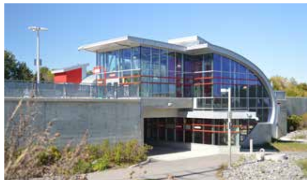
Ottawa Transitway: Queensway Station (top), Longfield Station (bottom).
