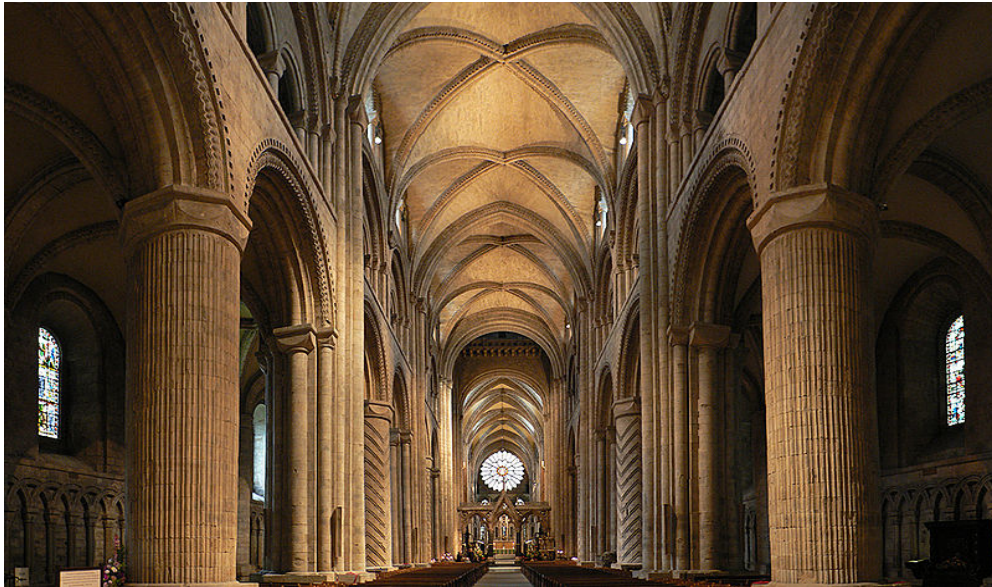
Figure 4. Nave, Durham Cathedral, England. 1093 – 1130.
