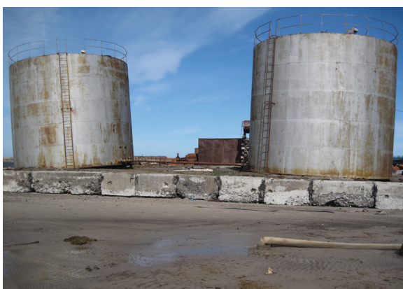
These images from July 2010 show the effects of permafrost deterioration on structures at Amerderma airfield and ground collapse in the land nearby. Photos courtesy of Gerald V. Frost.
