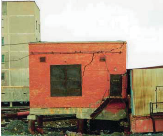
The thawing of ice-rich permafrost around an underground utility line causes structural deformations in the residential area of Oganer near Norilsk (July 2003).
