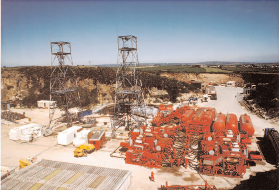
Figure 4.7 Major stimulation of Well RH15 at Rosemanowes in July 1985, 5,500m 3 at up to 265 L/s (100 bbl/min), surface pressure of 16 MPa (2,320 psi).
