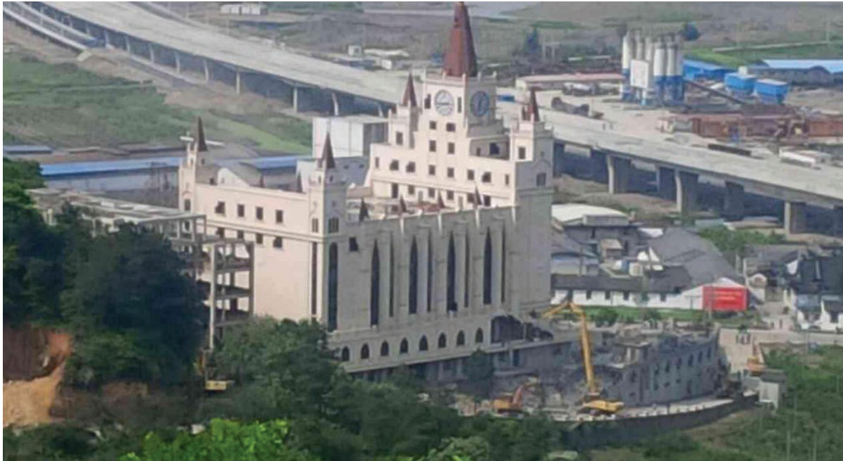
Sanjiang Cathedral, which belonged to an officially recognized church, in Zhejiang Province before and after its demolition in April 2015.
