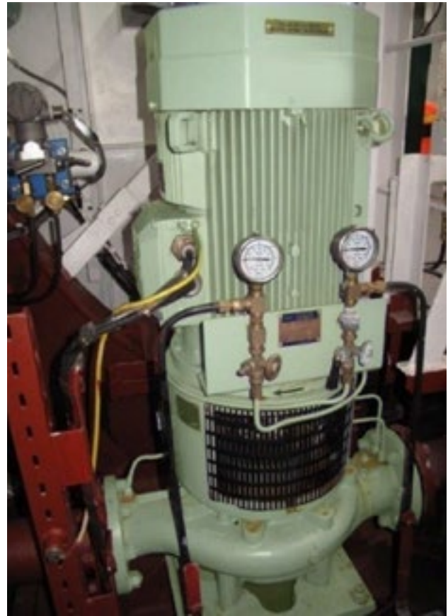
Figure: The sea water pump
