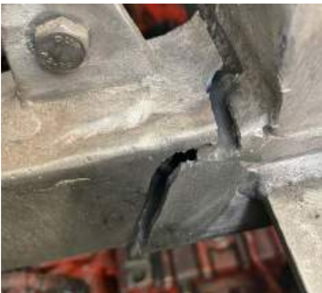
Figure 3: Fractured engine support
