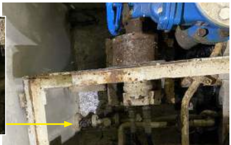
Figure: Fuel supply shut-off valve
