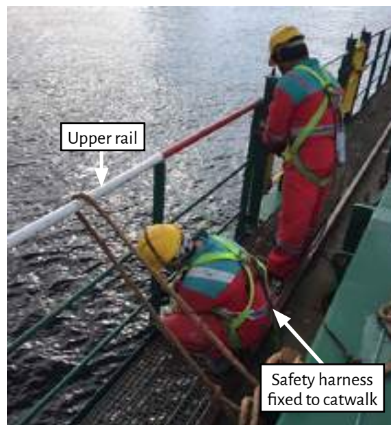
Figure 1: Bolts being removed from a section of upper rail
