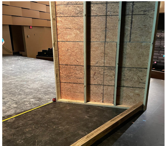
The Building of the Structure
