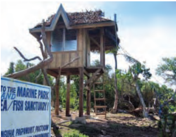
Marine sanctuary guard house used in law enforcement in the Philippines; it was erected with support from the community and IPOPCORM.
