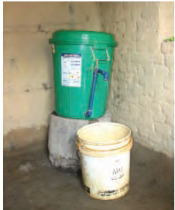
Arsenic-biosand filters made locally with plastic containers, gravel, sand and iron nails remove bacteria and arsenic from drinking water in the Khata Corridor, Nepal, thereby improving community health.
