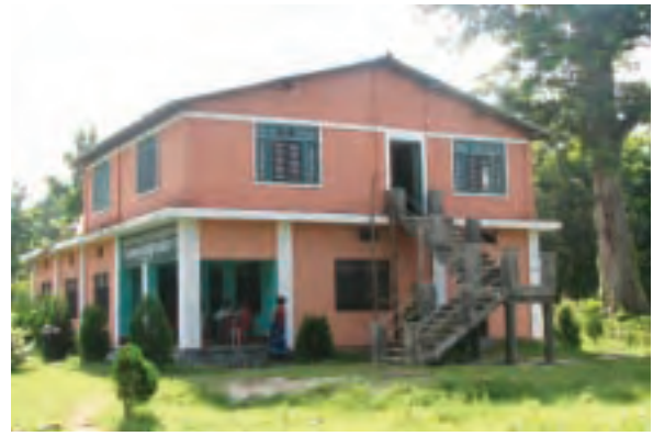
In the Khata Corridor in the Terai, Nepal, the Community Forest Coordination Committee runs a community clinic on the ground floor of its headquarters. Integrated project activities improve health, restore forests and wildlife, improve livelihoods, and generate revenue.
