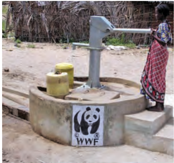
In the Kiunga Marine National Reserve in Kenya, hand pumps have been installed and wells have been covered in some villages to improve water quality.
