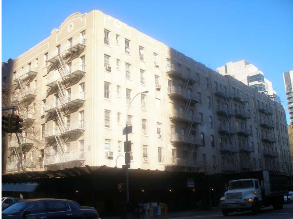
Amendment to City and Suburban Homes Company, First Avenue Estate 429 E. 64 th Street from the southeast showing the E. 64 th Street and York Avenue facades
