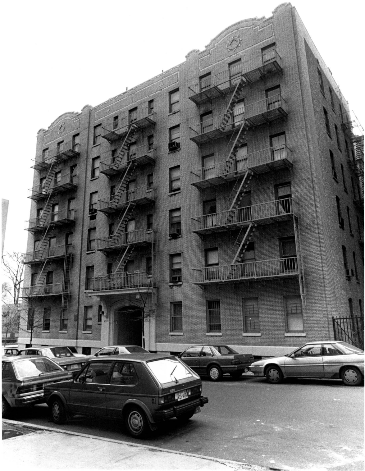
City and Suburban Homes Company, First Avenue Estate: 430 East 65 Street Photo Credit: Carl Forster
