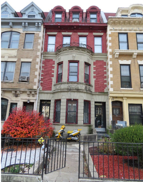
374-376 Parkside Avenue (Duplex A type) Bilge Kose, LPC, December 2022
