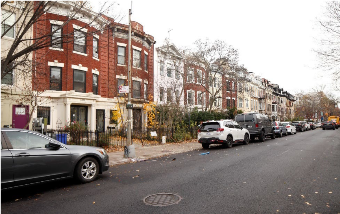
Parkside Avenue North Side Bilge Kose, LPC, December 2022
