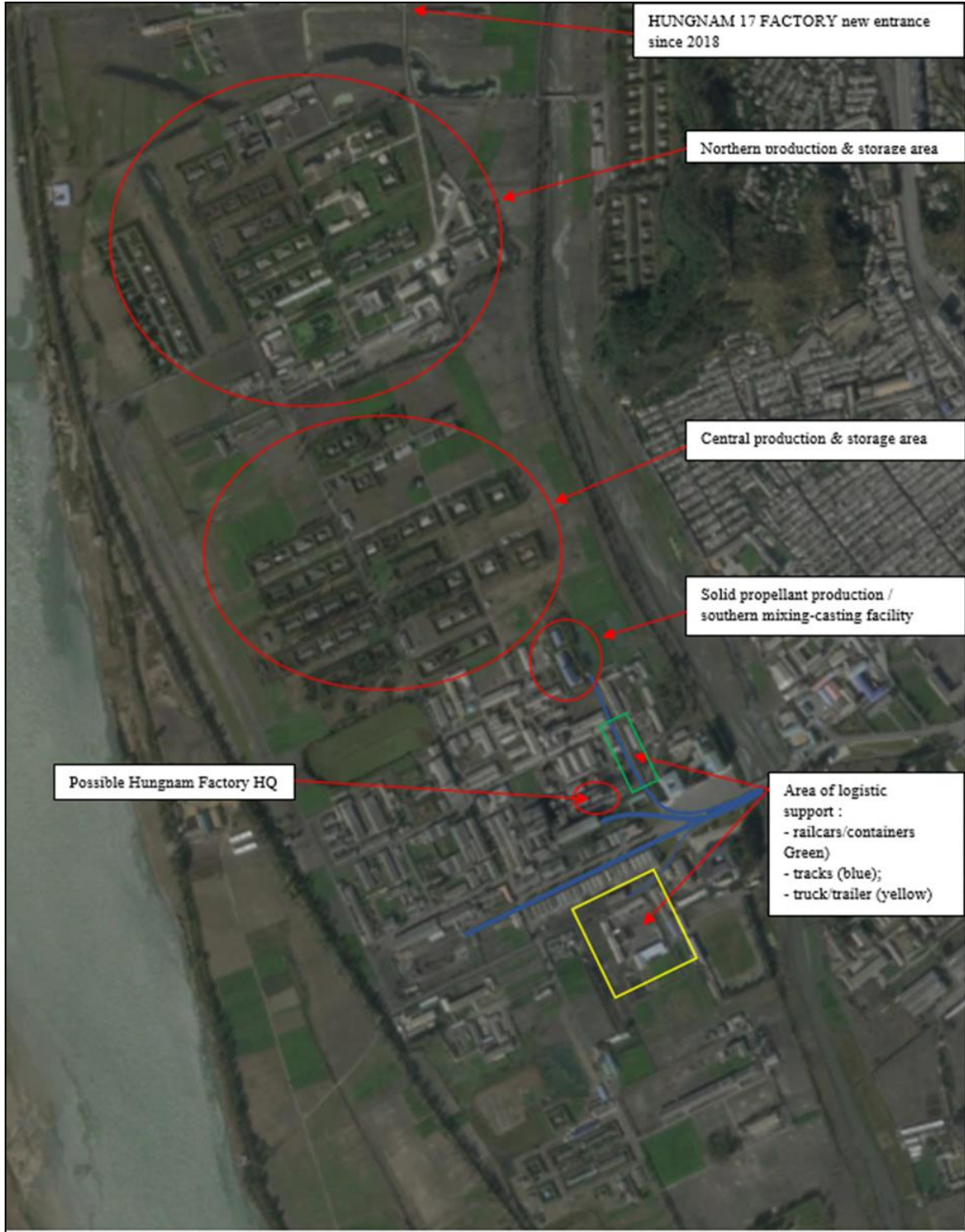
Figure 64.1: Overview of the Hungnam 17 Explosives Factory
