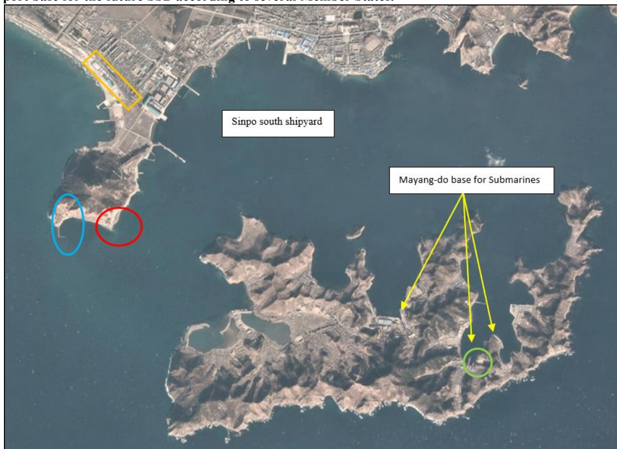
Figure 61.1: General view of Sinpo shipyard and Mayang-do base. This area could be used as a naval support base for the future SSB according to several Member States.
