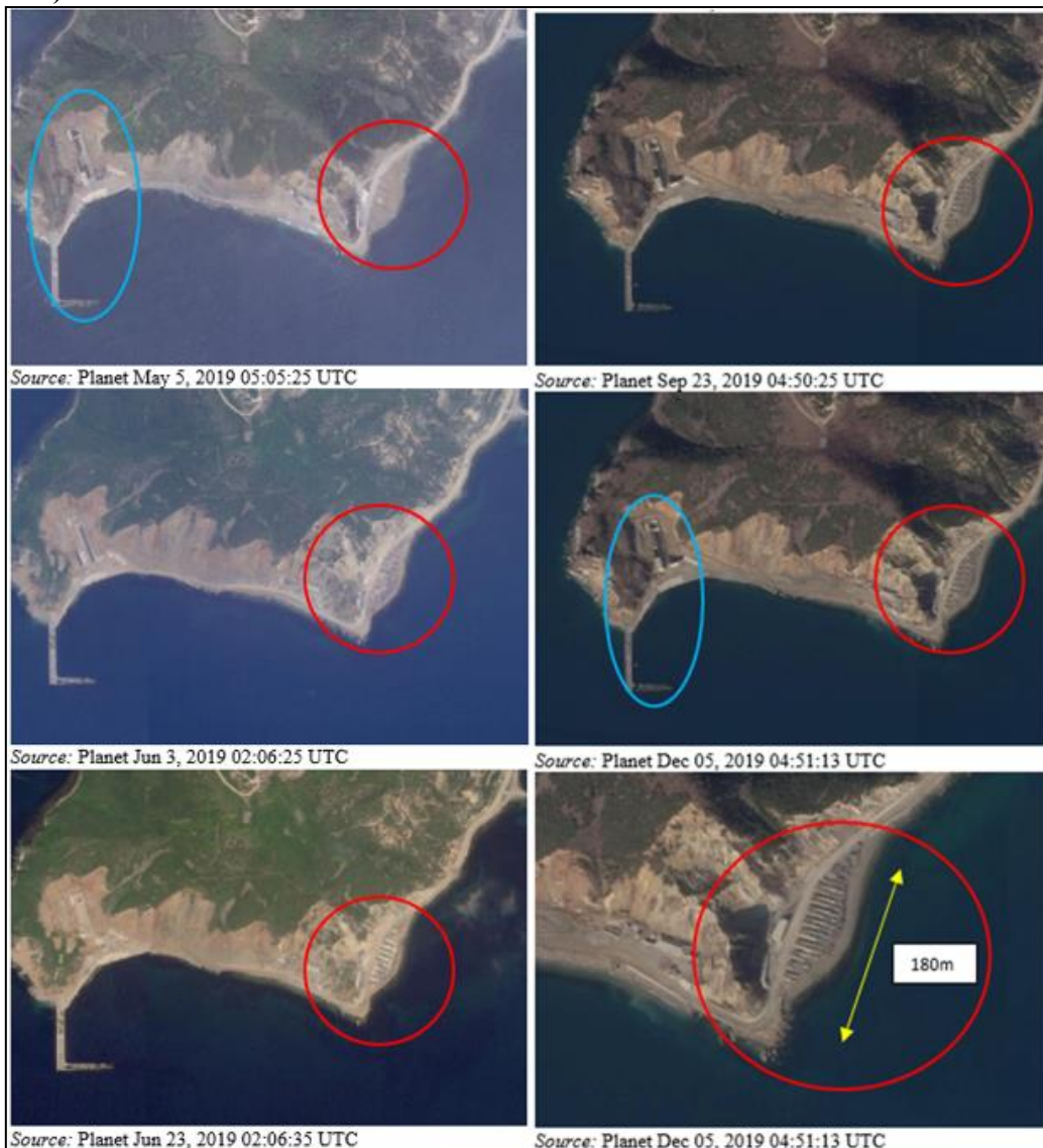
Figure 61.3: New infrastructure developments from May to Dec 2019 on the Sinpo peninsula (Figure red circle 40° 0'38.02"N 128° 9'21.50"E). Construction of the future underground submarine shelter (40° 0'42.23"N 128° 8'51.60"E) has slowed.
