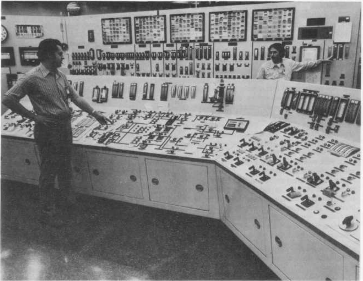
FIGURE 11-49. Visual Scan Necessary for Operator (on Left) Controlling Makeup To Monitor Makeup Flow (Operator on Right)
