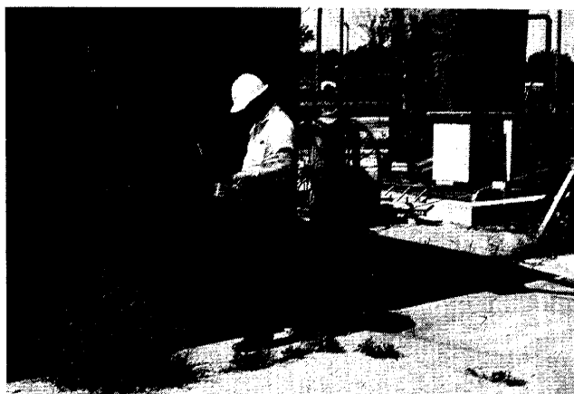
An NRC Region III radiation specialist performs a radiation survey in connection with the decontamination and dismantling of the Kerr-McGee thorium plant at West Chicago, Illinois. Such radiation surveys are used in determining alternative methods of decommissioning.
