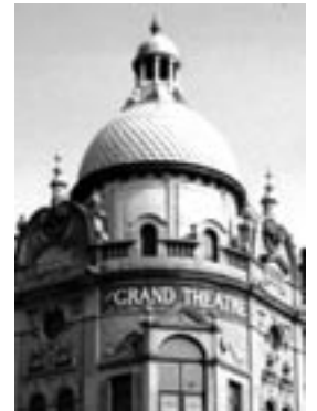
Chapter 4: Lifting Quality in the Built Environment
