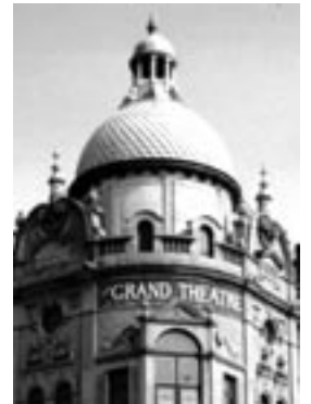
Chapter 4: Lifting Quality in the Built Environment
