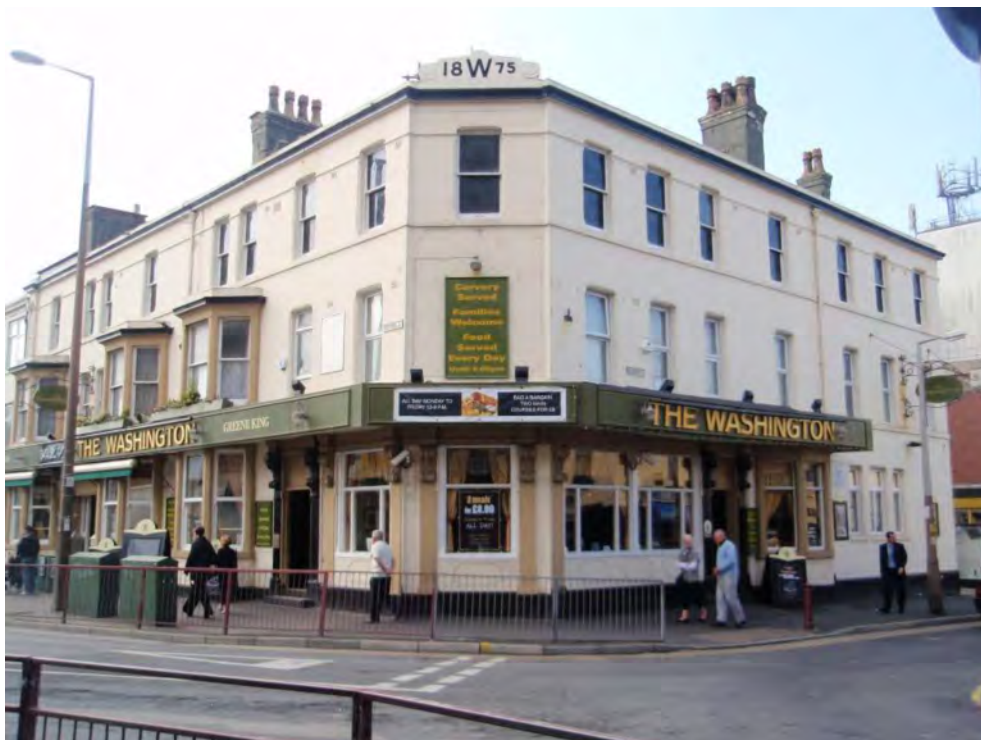
Fig. 79: The Washington, corner of Wood Street and Topping Street
