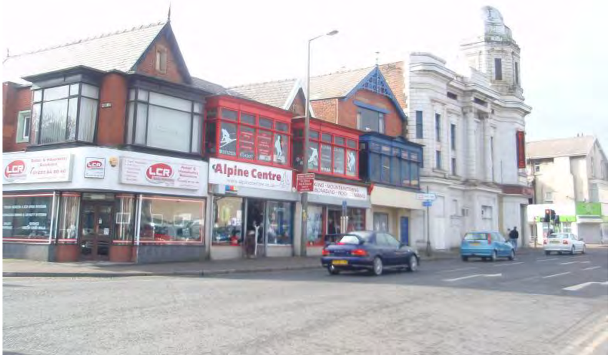
Fig. 107: Nos 193-197 Church Street, next to Riley's Pool Hall
