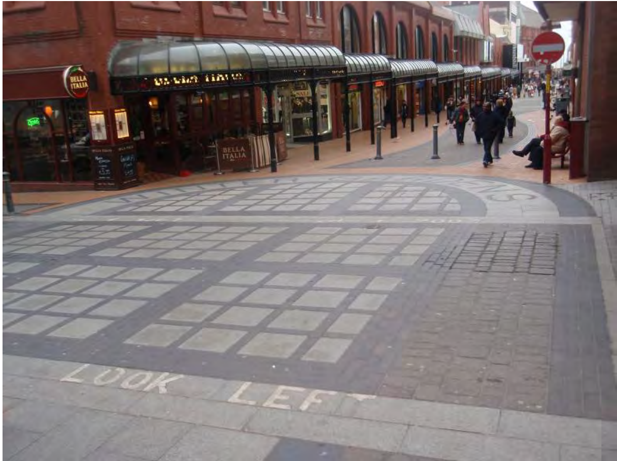
Fig. 34: Various non-traditional street surfaces to Victoria Street
