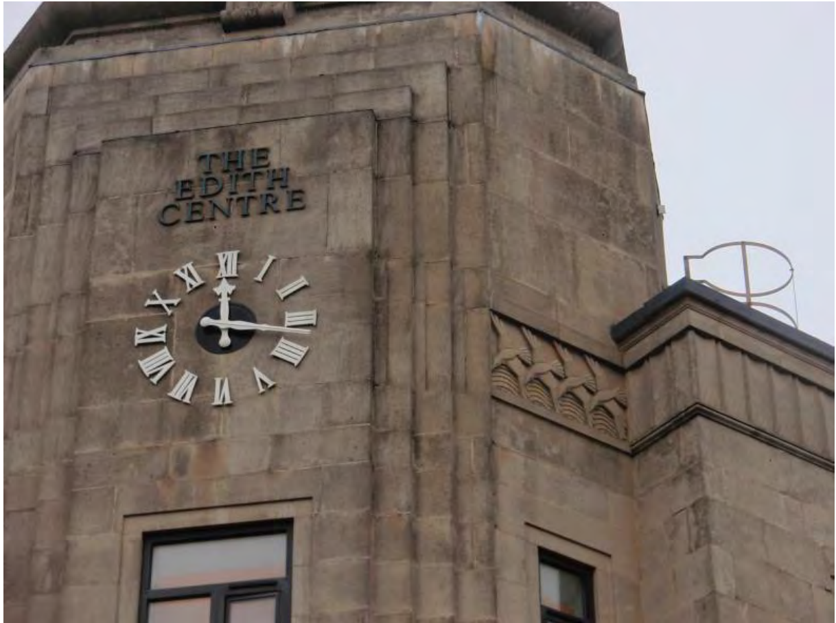
Fig. 42: Detail of the corner tower of the Edith Centre, to the junction of Bank Hey Street and Albert Road
