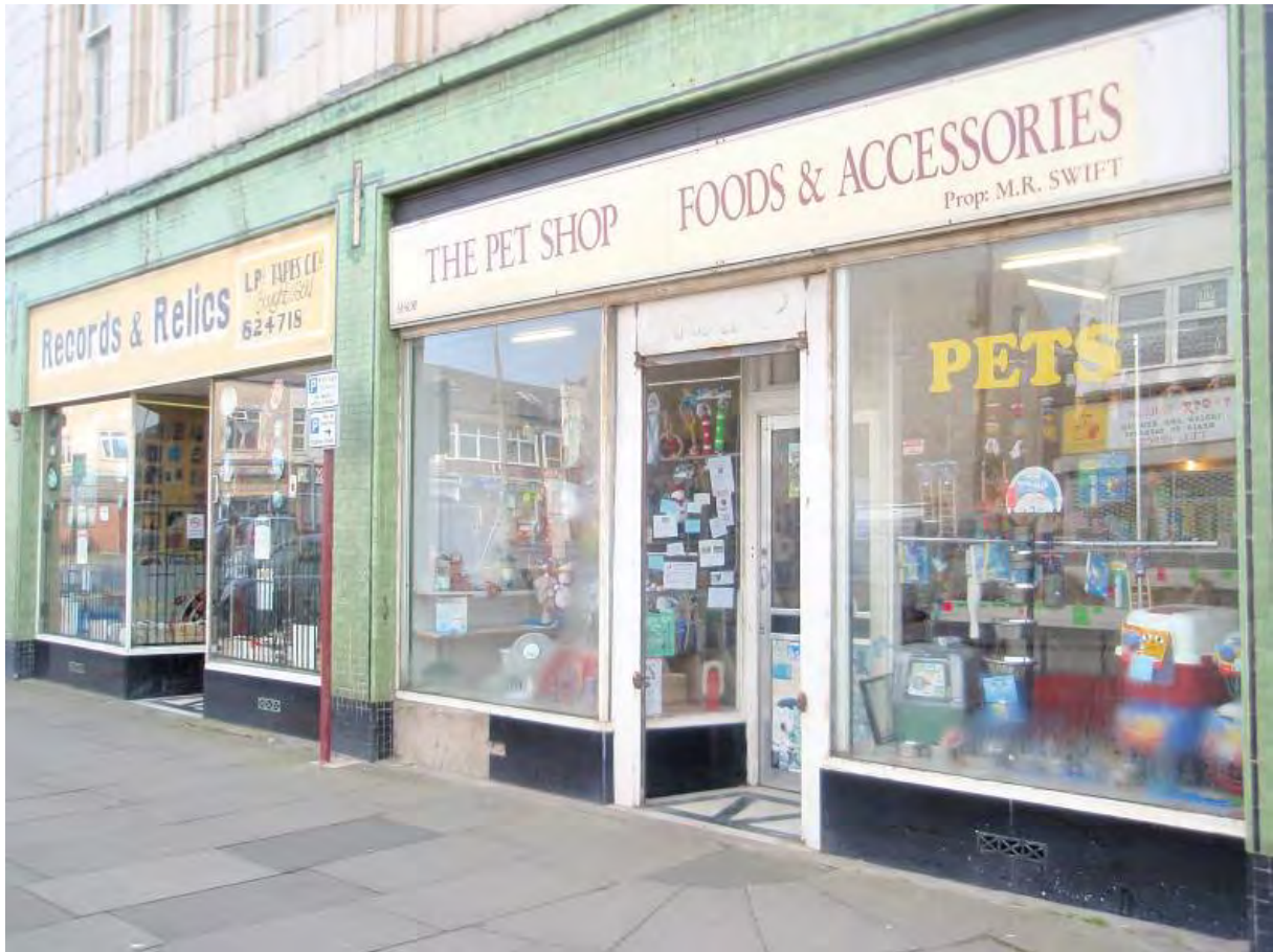
Fig.23: Shopfronts to Cauce Street
