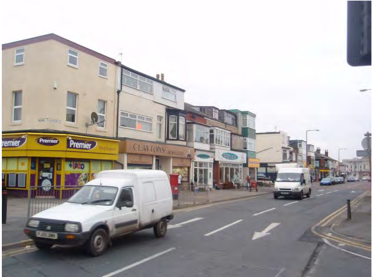
Fig. 109: The east side of Cookson Street from the north
