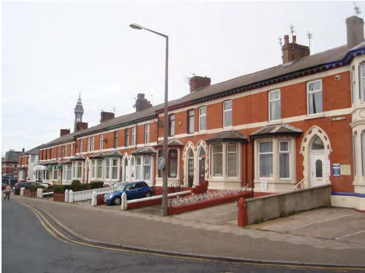
Fig.96: Nos 136-154 Albert Road
