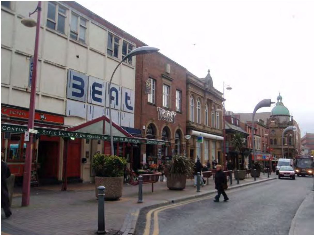
Fig. 65: East side of Corporation Street, looking south
