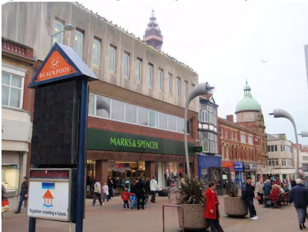
Fig. 58: Looking west along the south side of Church Street
