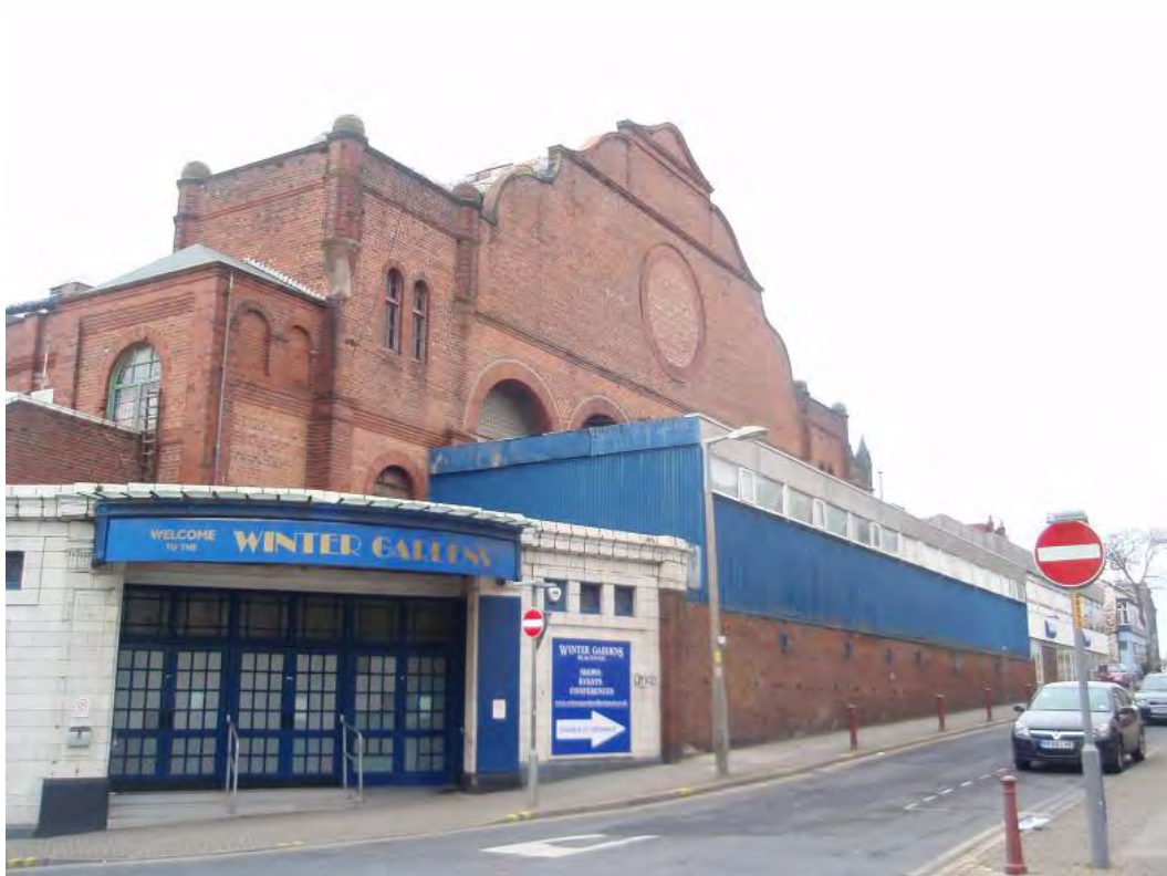
Fig. 113: The east elevation of the Winter Gardens complex and corner entrance
