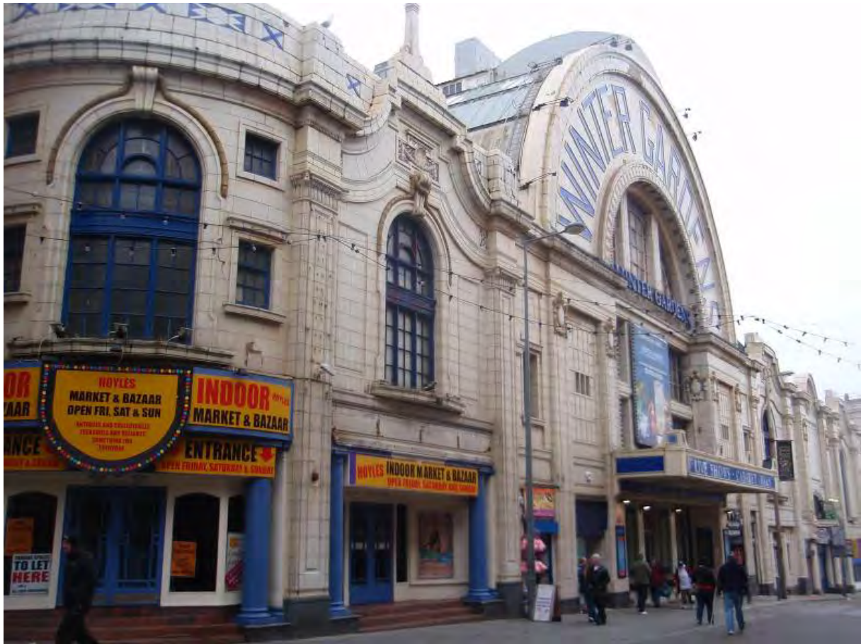
Fig. 17: Faience to the Coronation Street elevation of the Winter Gardens, re-faced in 1930
