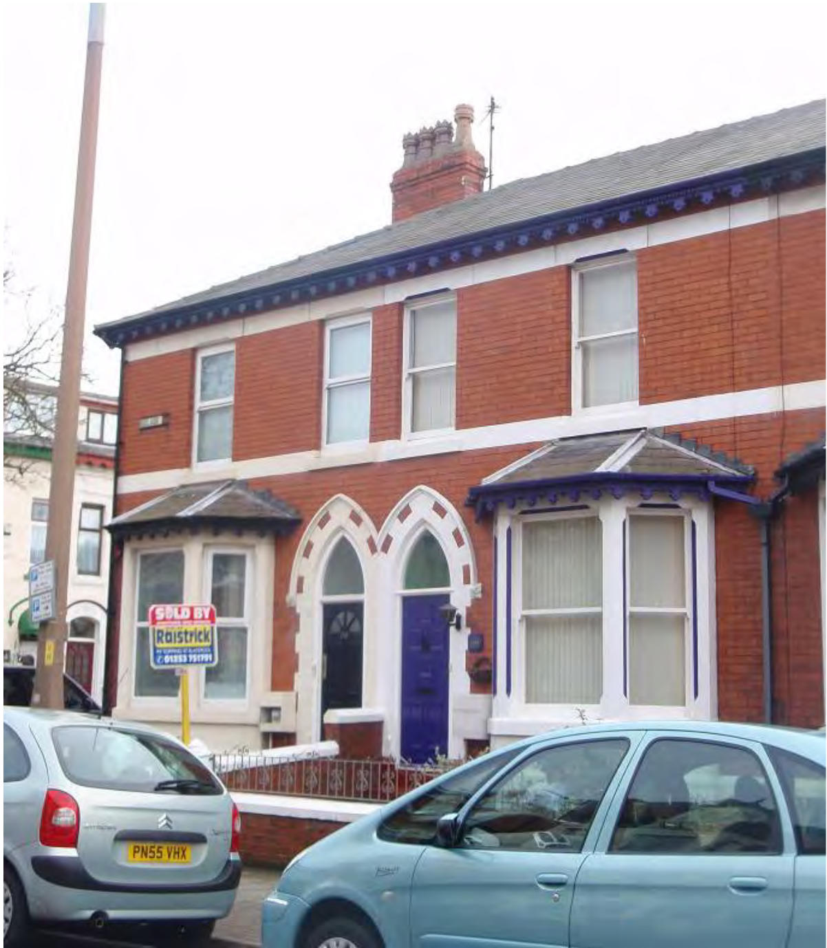
Fig. 19: End of terrace on Adelaide Street, canted bay windows with timber sash windows and panelled door on the right and uPVC casements on the left.
