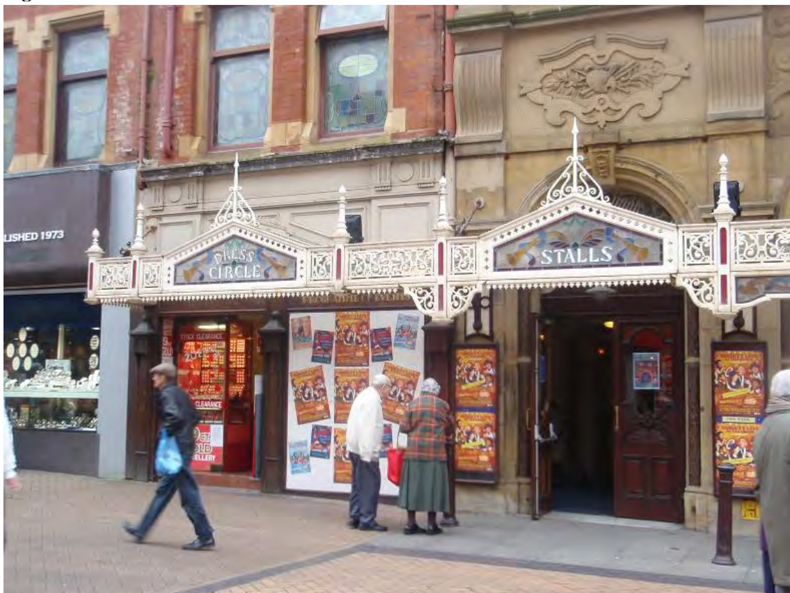
Fig. 27: Canopies to Grand Theatre entrance
