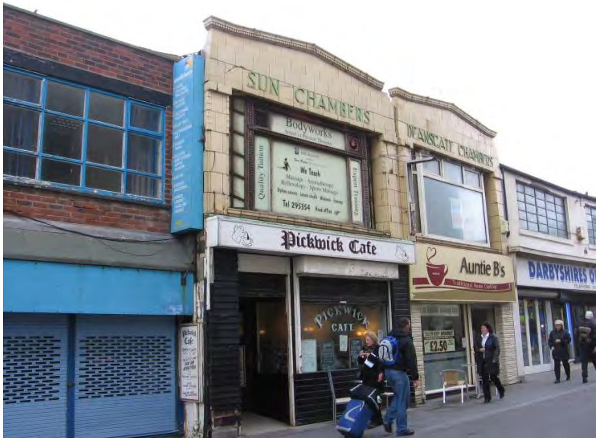
Fig. 40: Sun Chambers and Deansgate Chambers on Deansgate
