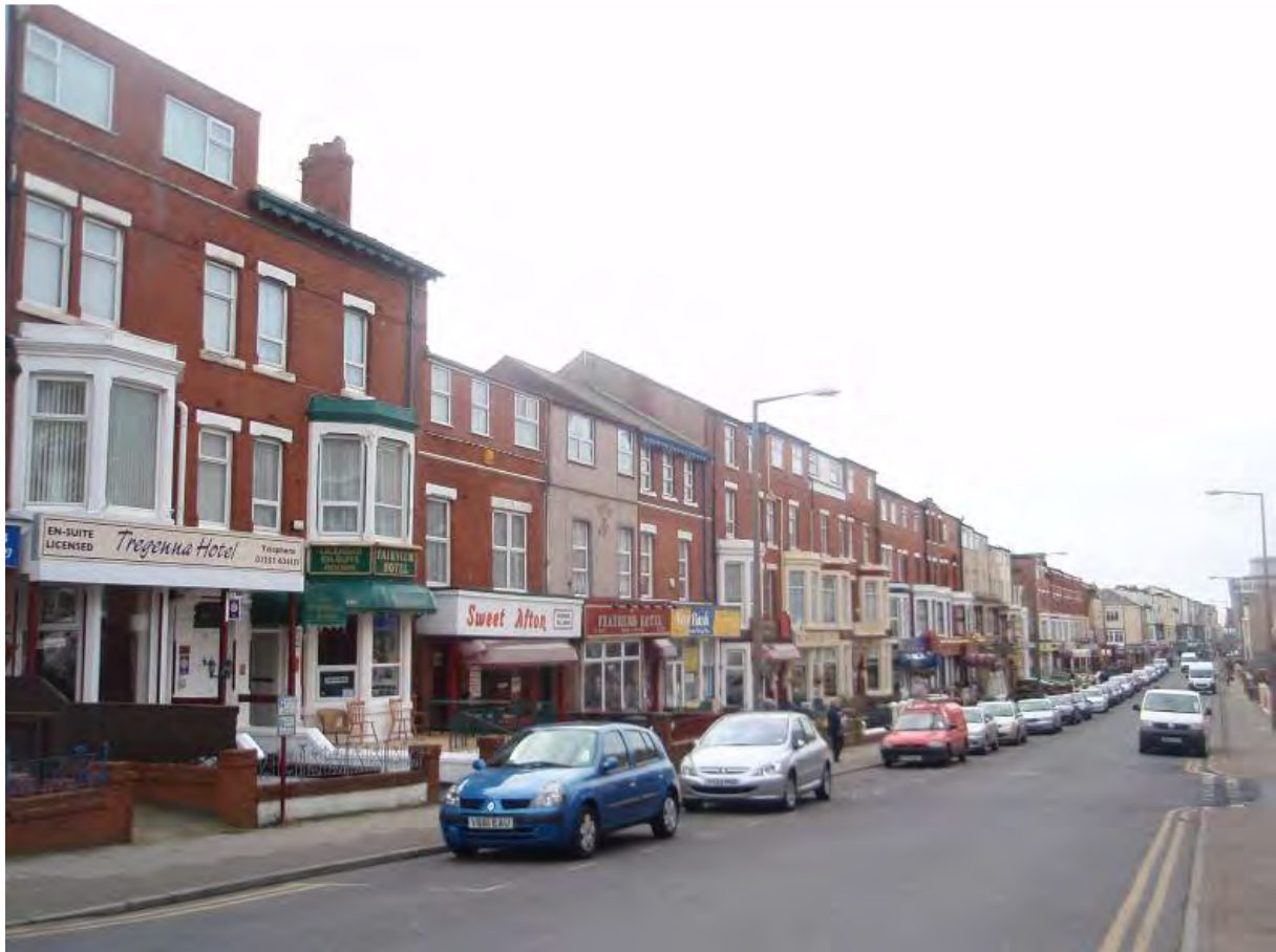
Fig. 95: Nos. 73-117 Albert Road from the east
