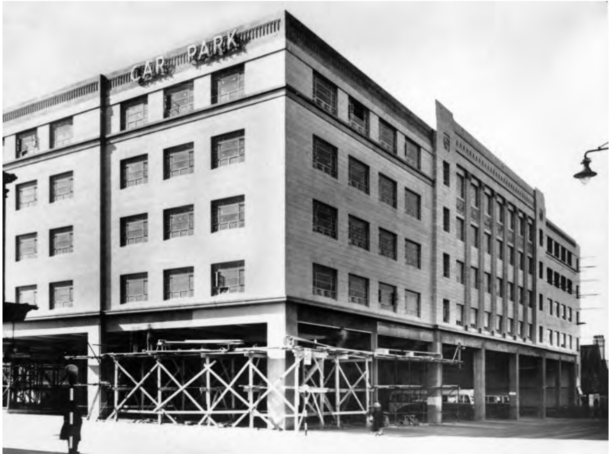
Fig. 8: Talbot Road car park shortly before completion in 1939 (reproduced with permission of Ted Lightbown)
