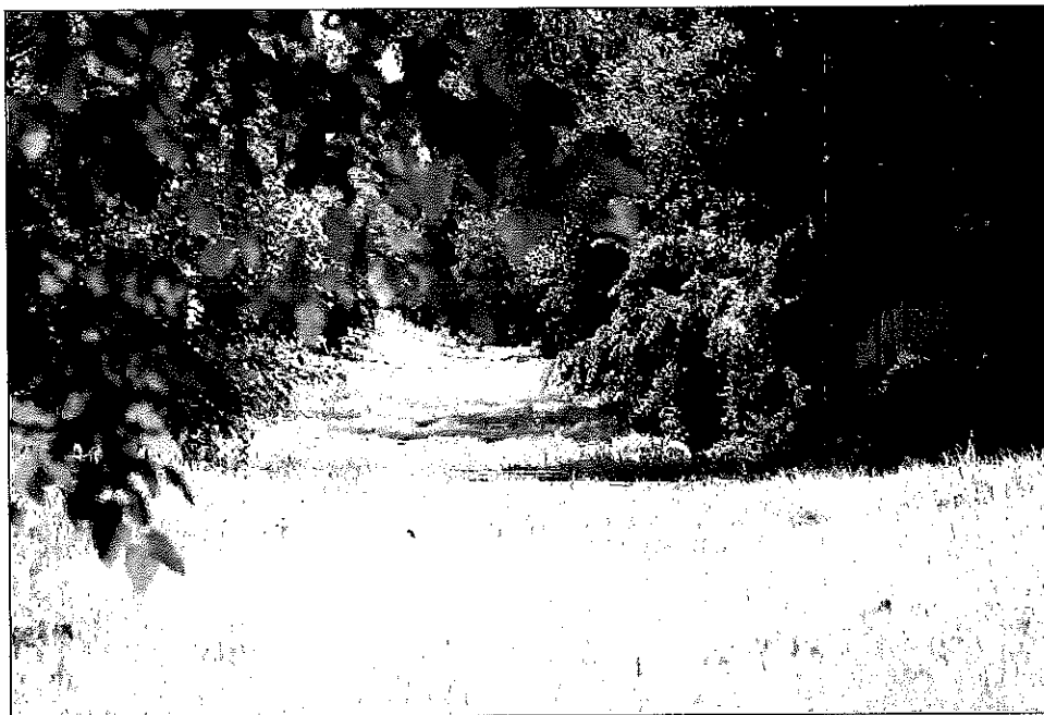
Image 2. View of Segment 3 looking south near intersection of Sullivan Drive and Lembeck Avenue following the original right of way route of the Morris Canal.
