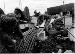
Photo 6 Laying electrical cables in ladder racking during the further development of the Project
