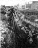
Photo 5 The Stanley water main from Moody Brook treatment plant to Dairy Paddock reservoir. Dewatering in progress
