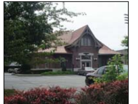
Above: View of historic Union Station on Frederica, now converted to offices
