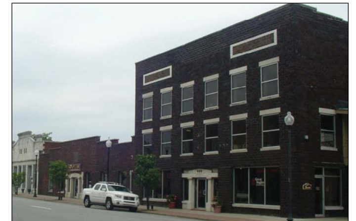
Existing historic buildings with potential for artists lofts and studios.
