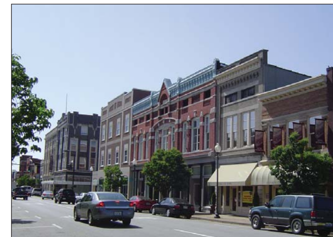
Existing facades on 2nd Street have architecturally harmonious facades
