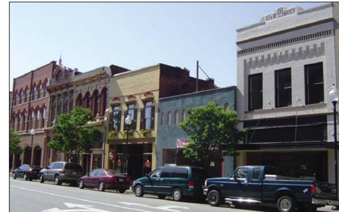
Section of 2nd Street with renovated storefronts
