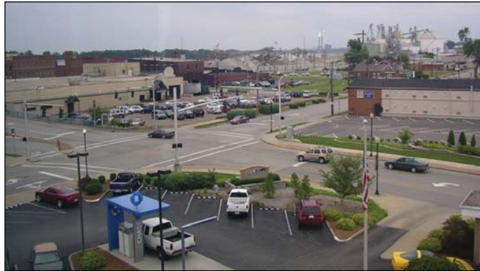
View of multi-story office buildings surrounded by surface parking characterizes the downtown core.
