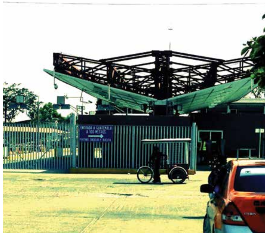
The recently built entry facility at Ciudad Hidalgo, Mexico. New biometric kiosks are inside.
