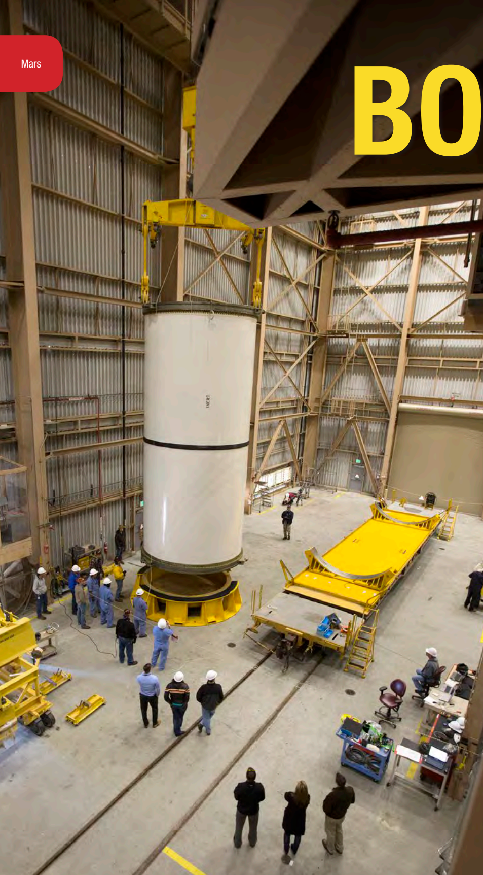
The first of two pathfinders, or test versions, of solid rocket booster segments for NASA's Space Launch System rocket was raised into the vertical position Feb. 25 and then lowered onto a test stand. Photo credit: NASA/Ben Smegelsky
