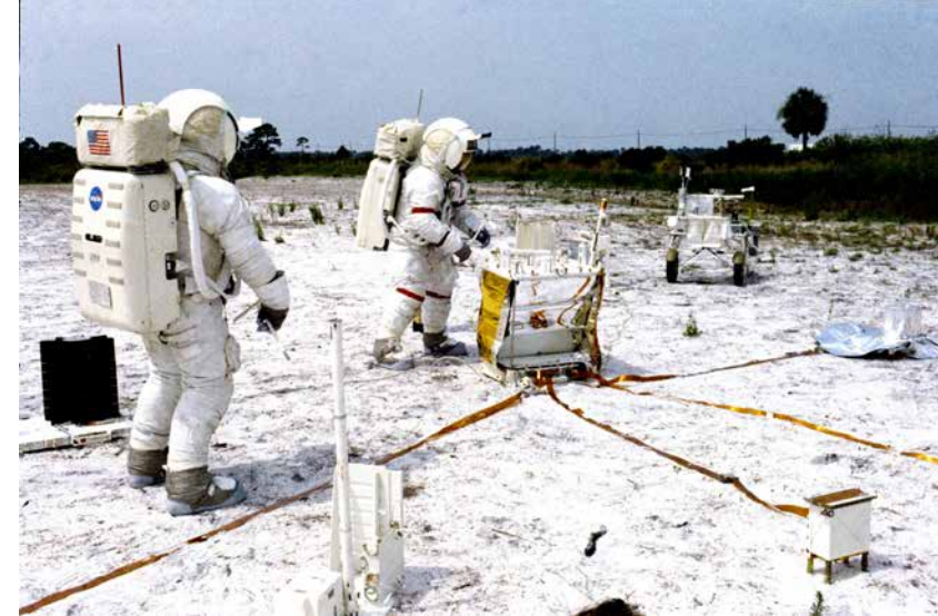
Edgar Mitchell, left, and Alan Shepard participate in lunar surface simulation training at Kennedy Space Center. They are deploying components of the Apollo Lunar Surface Experiments Package. Photo credit: NASA
