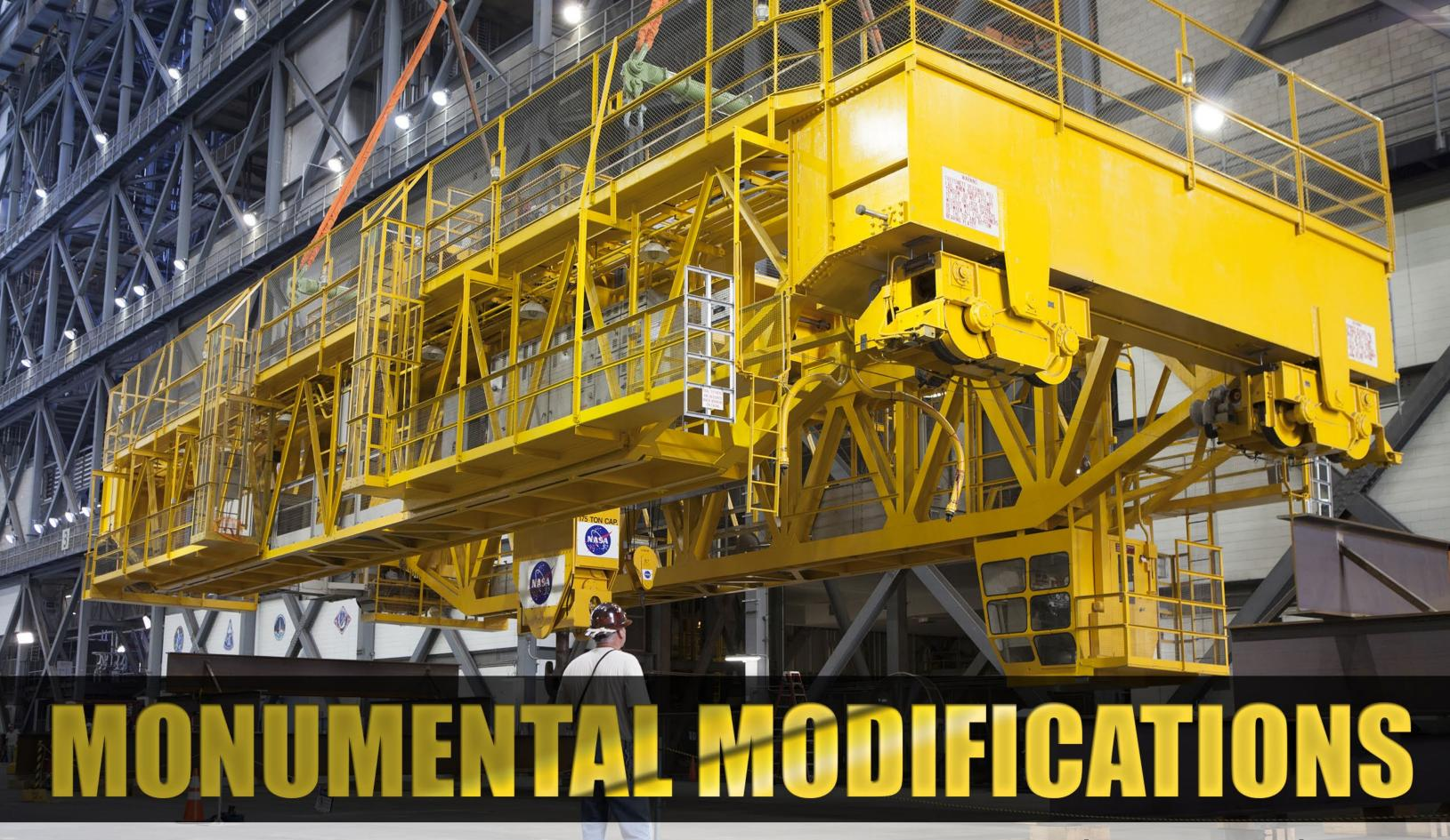
The 175-ton crane is lowered by crane Sept. 18 onto steel work stands on the transfer aisle floor of the Vehicle Assembly Building at Kennedy Space Center. Photo credit: NASA/Daniel Casper
