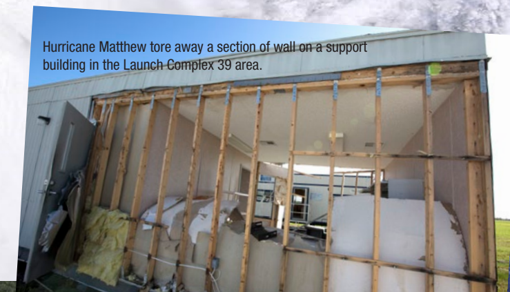
Siding damage caused by Hurricane Matthew is seen inside a support building in the Launch Complex 39 area.
