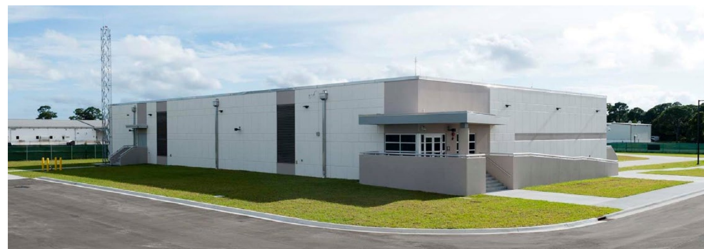
The Kennedy Data Center opened in October 2015. By consolidating multiple data centers into a single new one, Kennedy streamlined IT operations and improved efficiency. Photo credit: NASA
