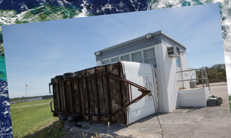
A damaged construction trailer and several pieces of associated debris, aftermath of Hurricane Matthew, are seen near the Mobile Launcher in the Launch Complex 39 area
