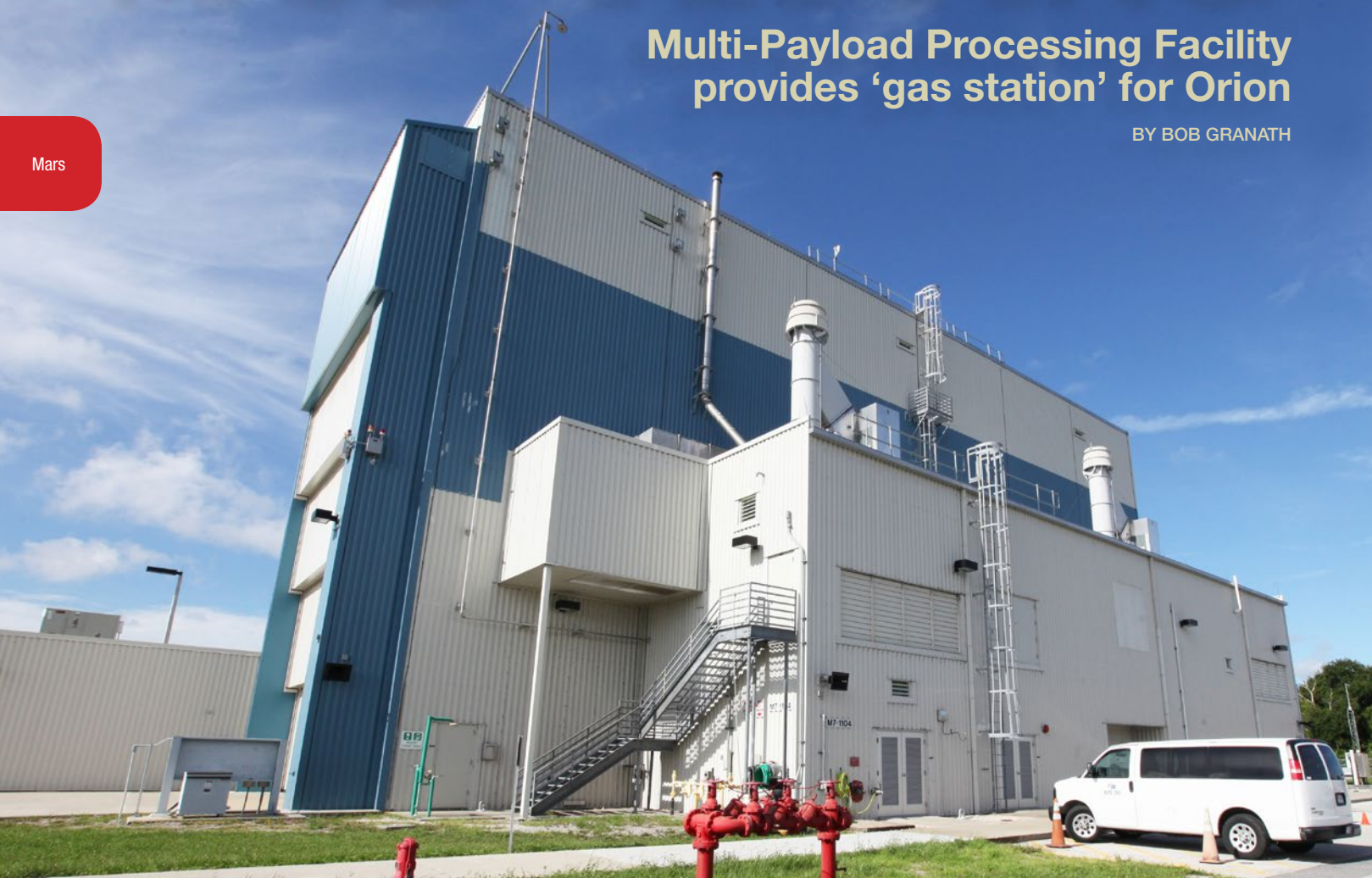
The 19,647-square-foot Multi-Payload Processing Facility is where Orion will receive its flight load of propellant, high pressure gasses and coolant. After years of design work, state-of-the-art equipment now is being tested. Photo credit: NASA/Ben Smegelsky
