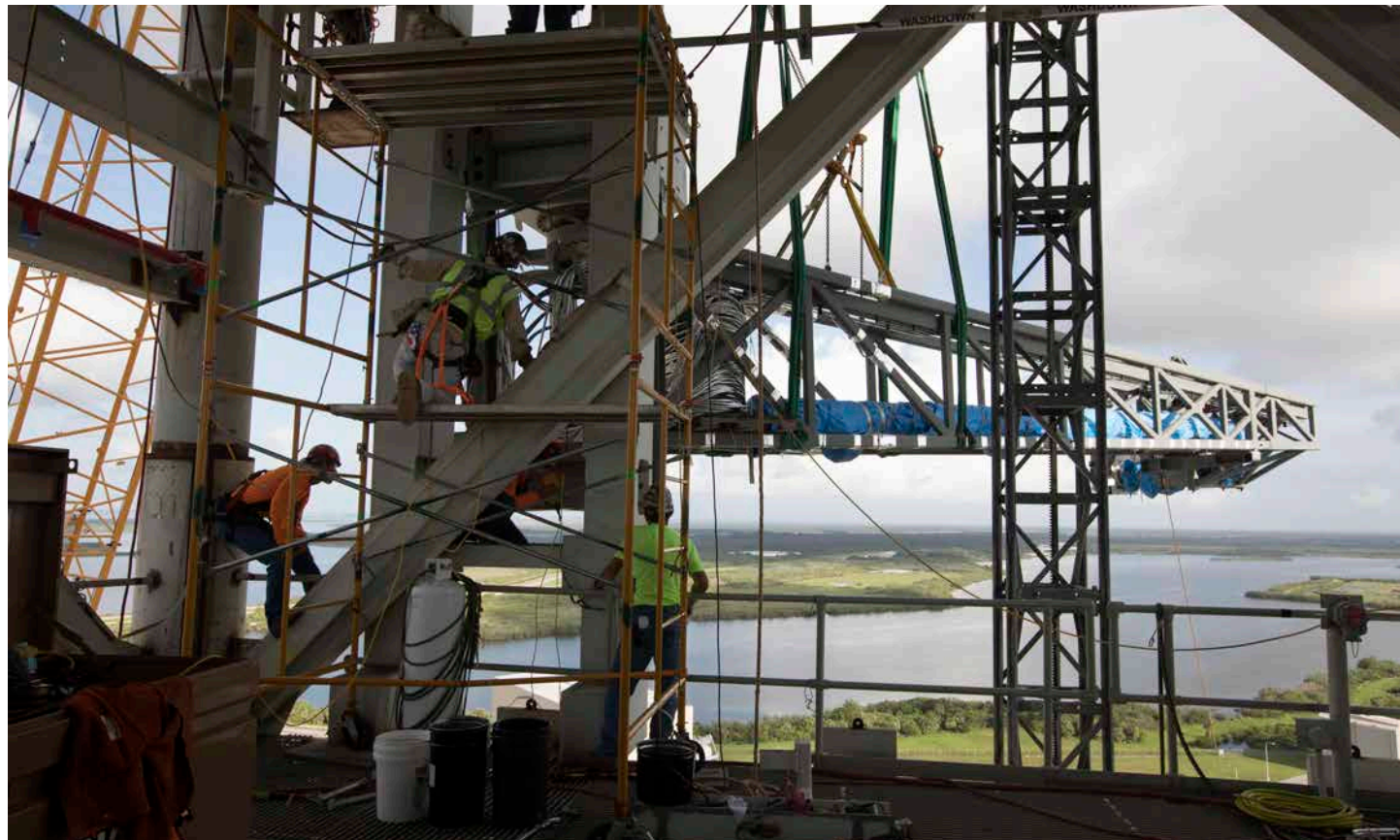
Technicians install the Core Stage Forward Skirt Umbilical on the mobile launcher. Photo credit: NASA/Kim Shiflett
