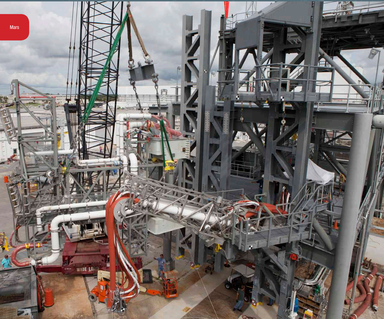
A view from above shows a heavy-lift crane attached to the Interim Cryogenic Propulsion Stage Umbilical at the Launch Equipment Test Facility, or LETF, at Kennedy Space Center. Photo credit: NASA/Glenn Benson
