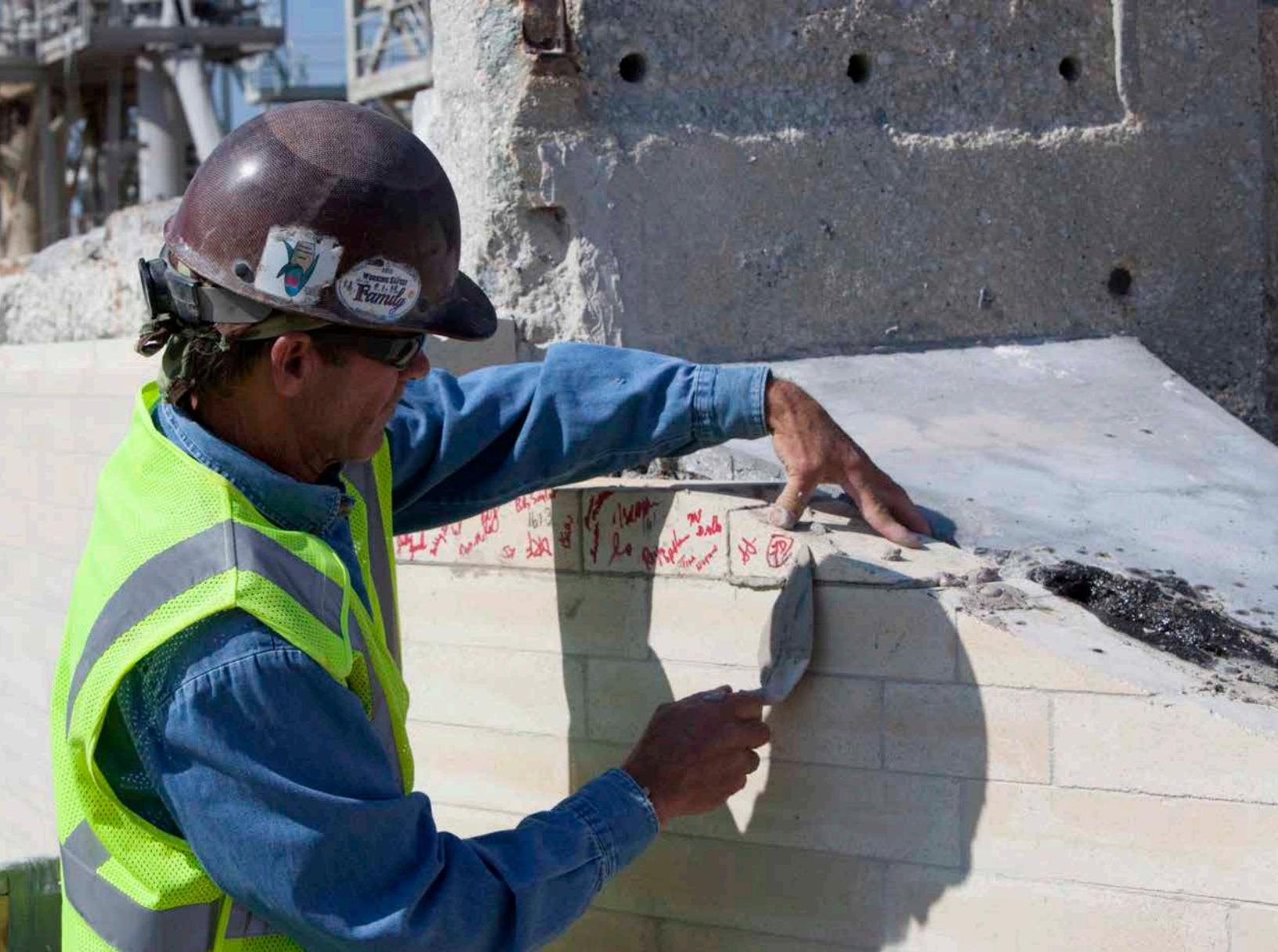
Jimmy Saylor, a mason with Reintjes Services, a subcontractor to JP Donovan, installs the final brick on the north side of the flame trench wall at Launch Complex 39B at Kennedy Space Center. Photo credit: NASA/Leif Heimbold
