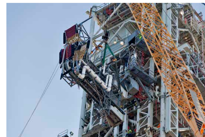
A heavy-lift crane and rigging lines are used to lift the Interim Cryogenic Propulsion Stage Umbilical high up for installation on the tower of the mobile launcher on March 16, 2018, at NASA's Kennedy Space Center. Photo credit: NASA/Ben Smegelsky
