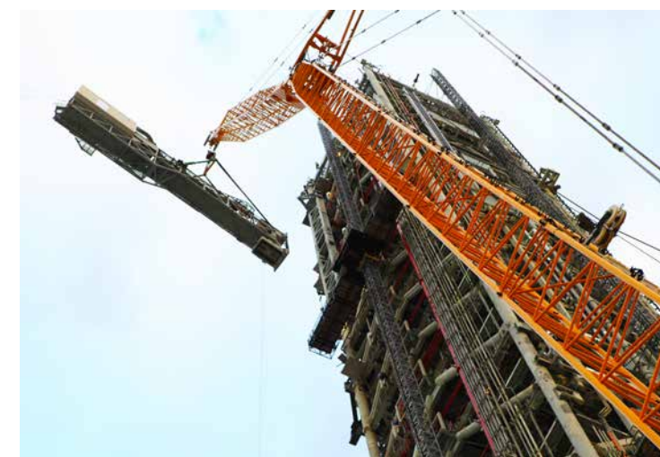
A crane lifts the Orion crew access arm so it can be attached to the mobile launcher at NASA's Kennedy Space Center. The crew access arm is designed to rotate from its retracted position and line up with Orion's crew hatch. The arm will provide entry and emergency egress for astronauts and technicians into and out of the Orion spacecraft. Photo credit: NASA/Bill White
