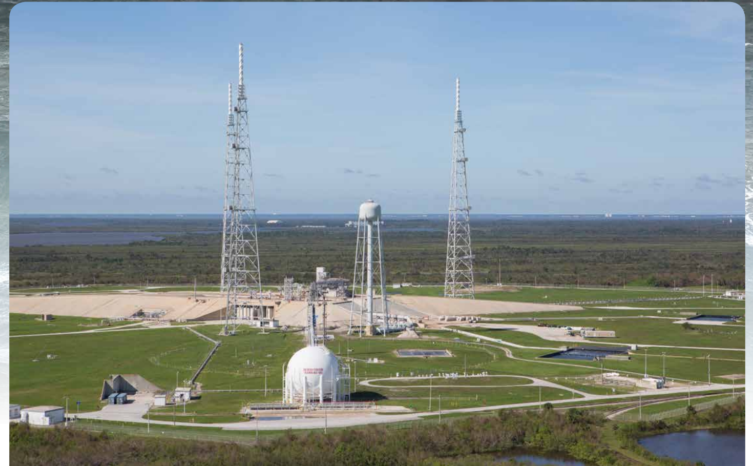
Launch Complex 39B is seen during an aerial survey of NASA's Kennedy Space Center in Florida on Oct. 8, 2016. The survey was performed to identify structures and facilities that may have sustained damage from Hurricane Matthew as the storm passed to the east of Kennedy on Oct. 6 and 7, 2016. Officials determined that the center received some isolated roof damage, damaged support buildings, a few downed power lines, and limited water intrusion. Beach erosion also occurred, although the storm surge was less than expected. NASA closed the center ahead of the storm's onset and only a small team of specialists, known as the Rideout Team, was on the center as the storm approached and passed. Photo credit: NASA/Cory Huston
