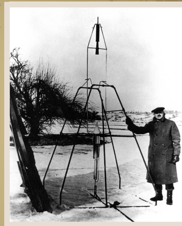
“I imagined how wonderful it would be to make some device which had even the possibility of ascending to Mars,” thought 17-year-old Robert Goddard in 1899. In the Massachusetts snow on March 16, 1926, he took the first step by developing and launching the world's first liquid propellant rocket. Photo credit: NASA
