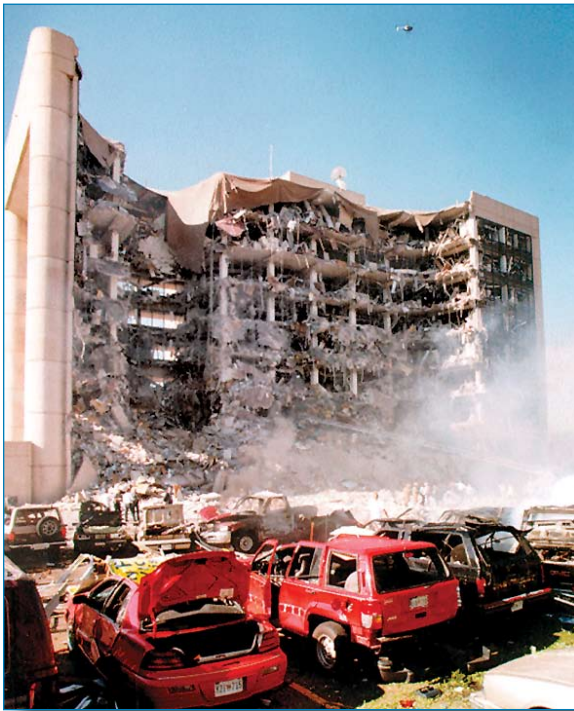
Figure 2-4 Alfred P. Murrah Federal Office Building
