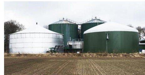
An example of Anaerobic digester
