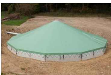
Examples of closed storage, with proper manure storage system
