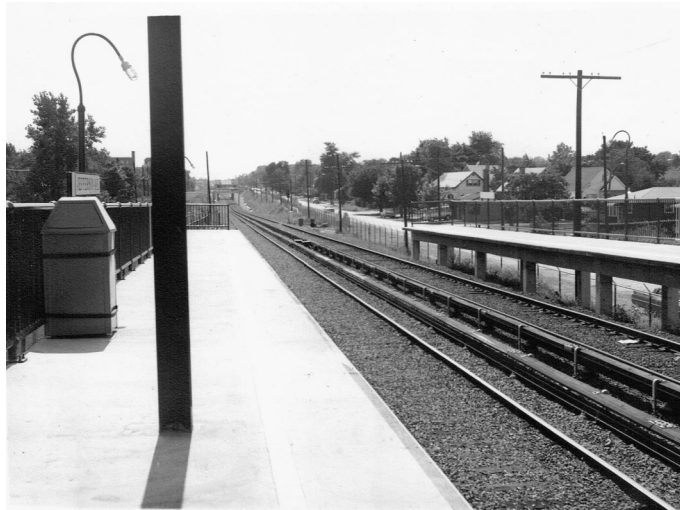
Jefferson Avenue, looking south, August 30, 1968. Larry Linder photograph
