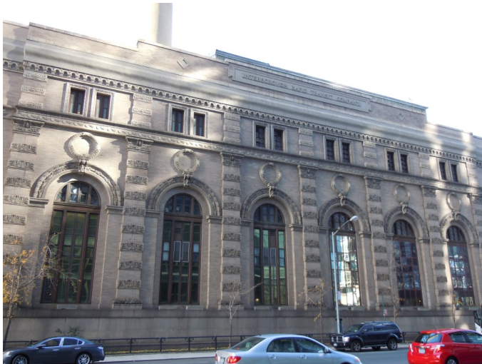
IRT Powerhouse, 11 th Avenue elevation eastern façade, December 3, 2011.
