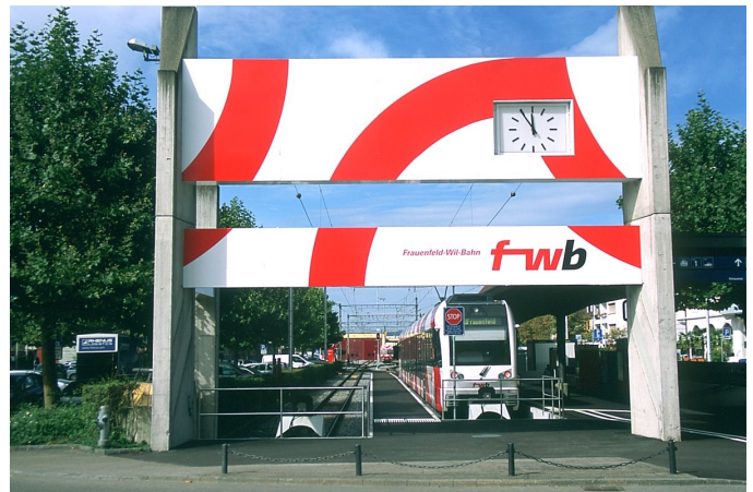
The Wil terminal of the Frauenfeld-Wil-Bahn, a few steps from the town's SBB station.
