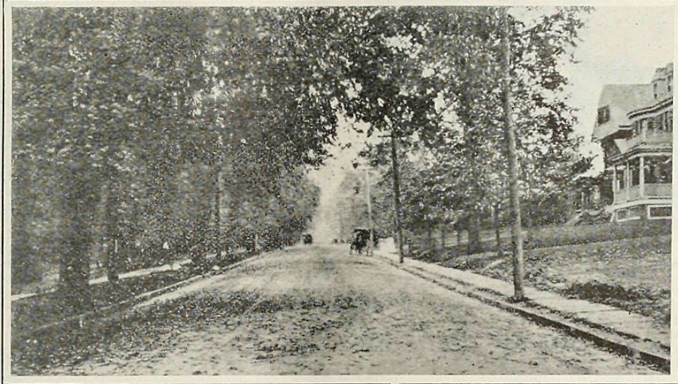
BARD AVENUE, WEST BRIGHTON.
