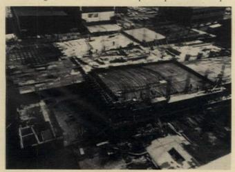
Tendons have been uncoiled on slab forms in foreground: in upper right, part of the concrete placement has been completed with additional concrete being pumped into place.
