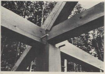
Typical joint (above) with wooden dowels; window casements (right) are used for intramural communication and reading.
