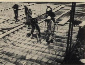
Pumping of concrete to form the slab. Temperature steel and tubes can be seen in place. Tendons are positioned in ribs between the tubes
