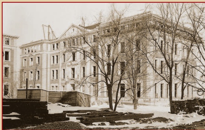
Havemeyer Hall under construction, 1897.
