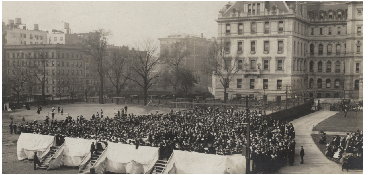
Construction and development has been a constant at the Cathedral. These images from 1916 depict the first breaking of the ground beginning work on the Nave. Photos: Diocesan Archives
