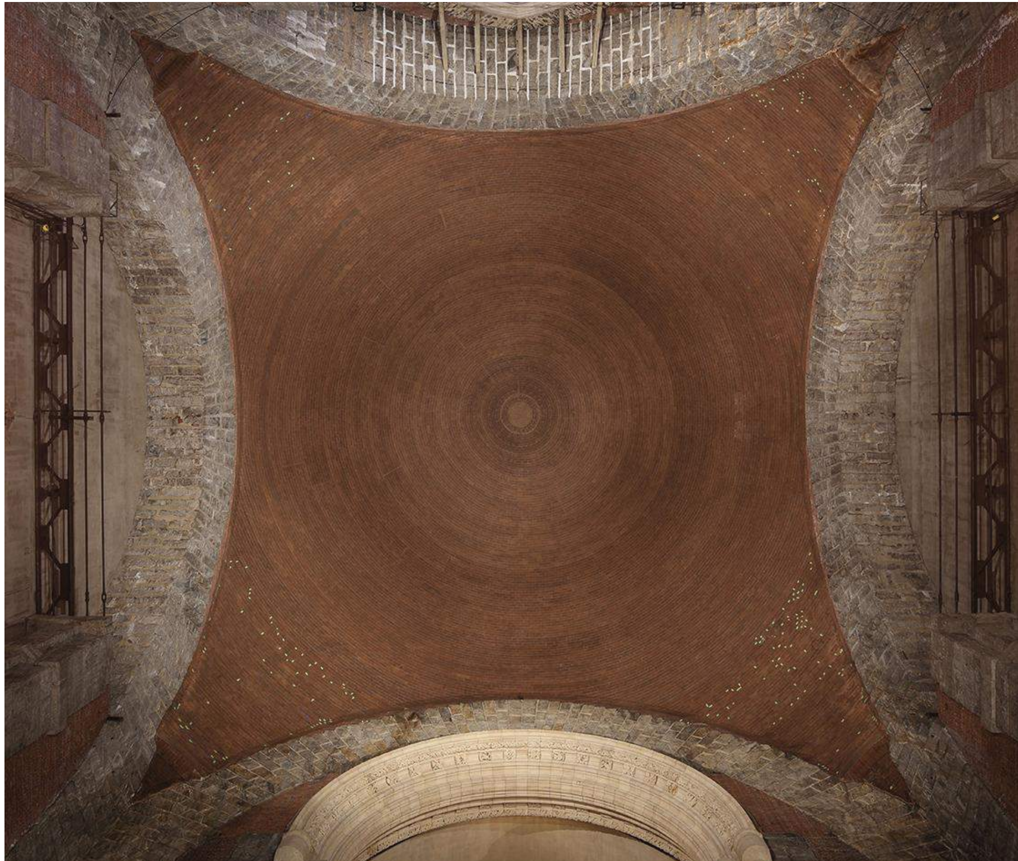
Photo of Guastavino Vault Underside, 2016
