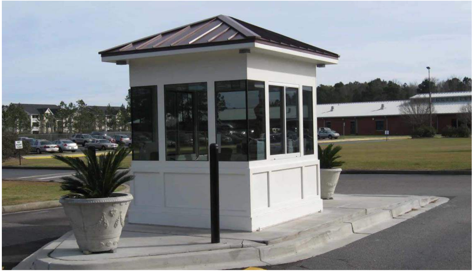
PROPOSED STANDING SEAM ROOF
