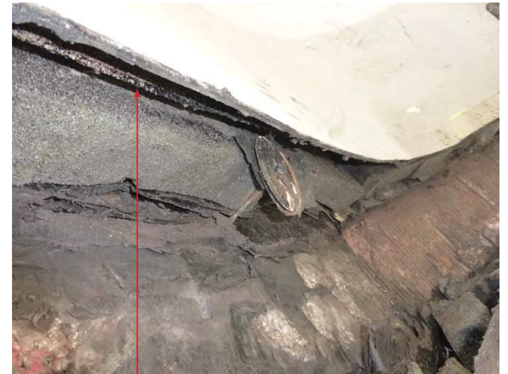
Outer waterproofing membrane is completely separated from Foamglass Insulation
