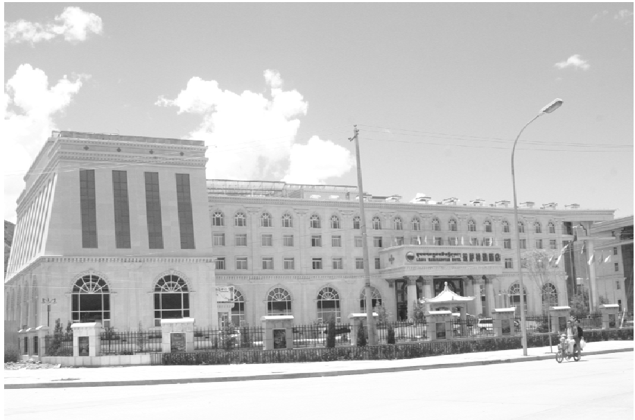
Hotel on former Kumbumthang land
