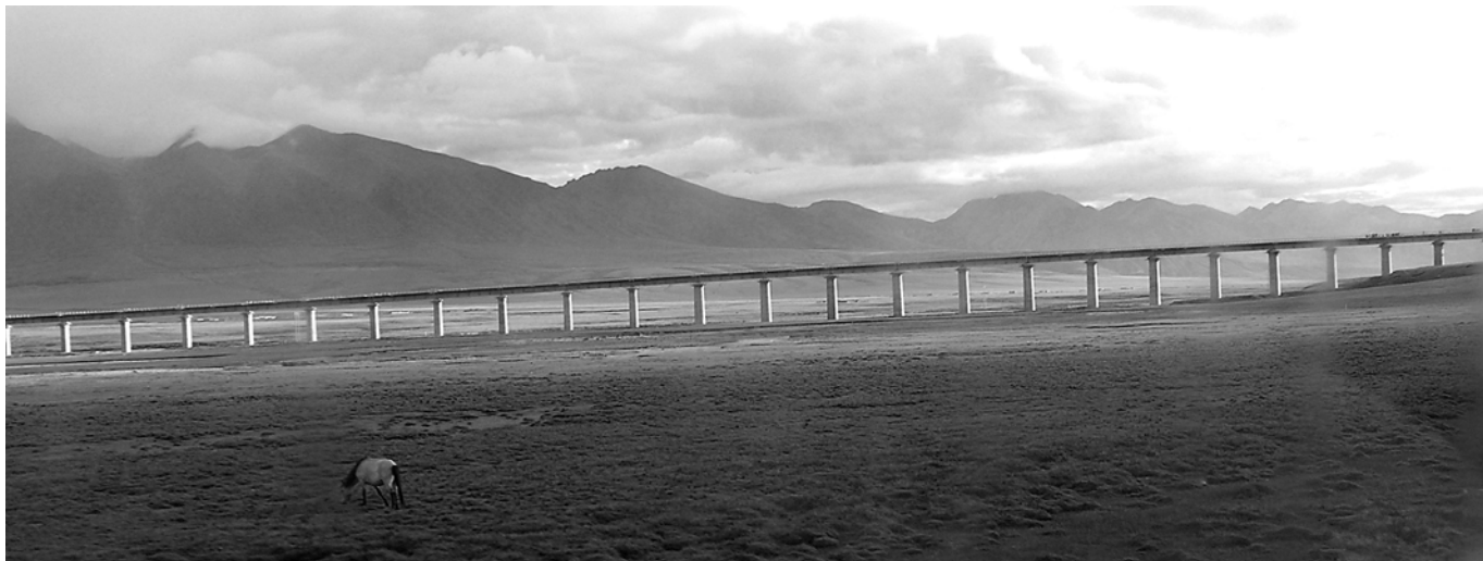
The track of the new railway from Gormo to Lhasa, partly elevated, cuts through the grasslands of the Tibetan plateau. Photo by Ran & Limi
