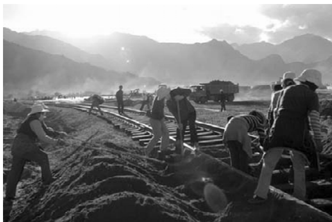
Tibetans performing menial jobs on a railway construction site.
