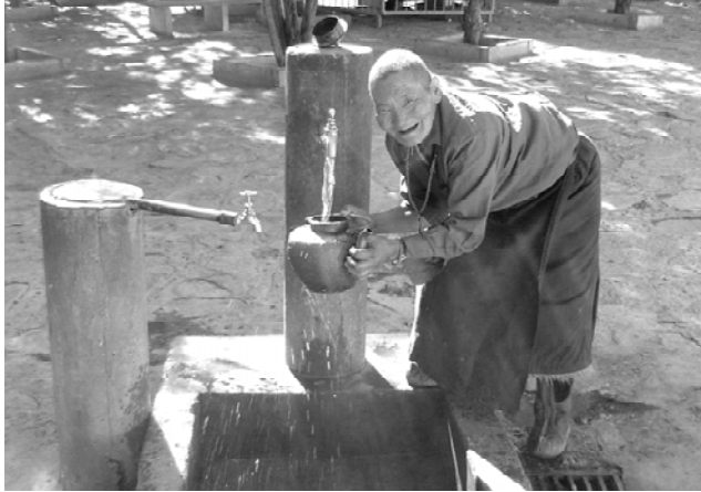
An elderly nun stoops to fill her water pot from a poorly-designed village tap, with no platform to rest heavy pots. Chronic back pain is a major health problem in Tibet.
