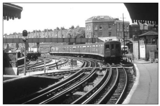
Left: Looking west from the west end of the eastbound platform at Westbourne Park with a six-car eastbound train of CO/CP Stock approaching station. Westbourne Park signal box can be seen on the right which closed on 13 March 1970 and the area converted automatic working. Note the flat crossing which, on the left, came from Crimea led sidinas and Portobello sidings on the Access to right. westbound Hammersmith & City Line was east of the
