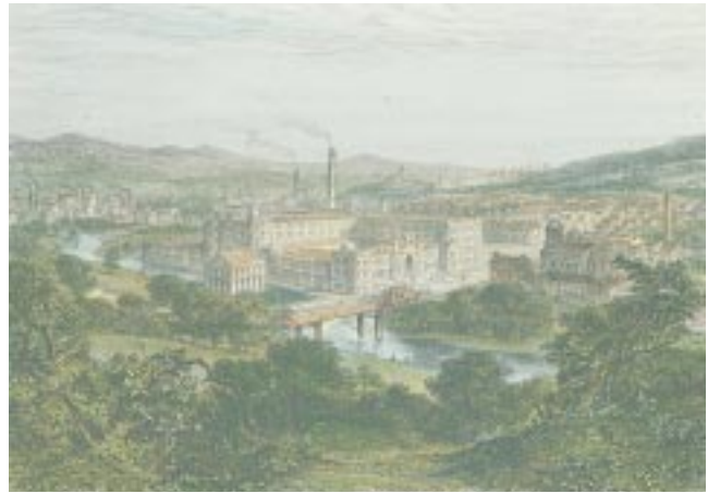
A NEW INDUSTRIAL TOWN. Cities and towns grew dramatically in Britain in the first half of the nineteenth century, largely as a result of industrialization. Pictured here is Saltaire, a model textile factory and town founded near Bradford by Titus Salt in 1851. To facilitate the transportation of goods, the town was built on the Leeds and Liverpool canals.
