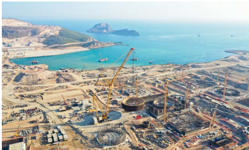
Reactors under construction at Akkuyu, Turkey. (Image: Akkuyu image bank, ROSATOM)
