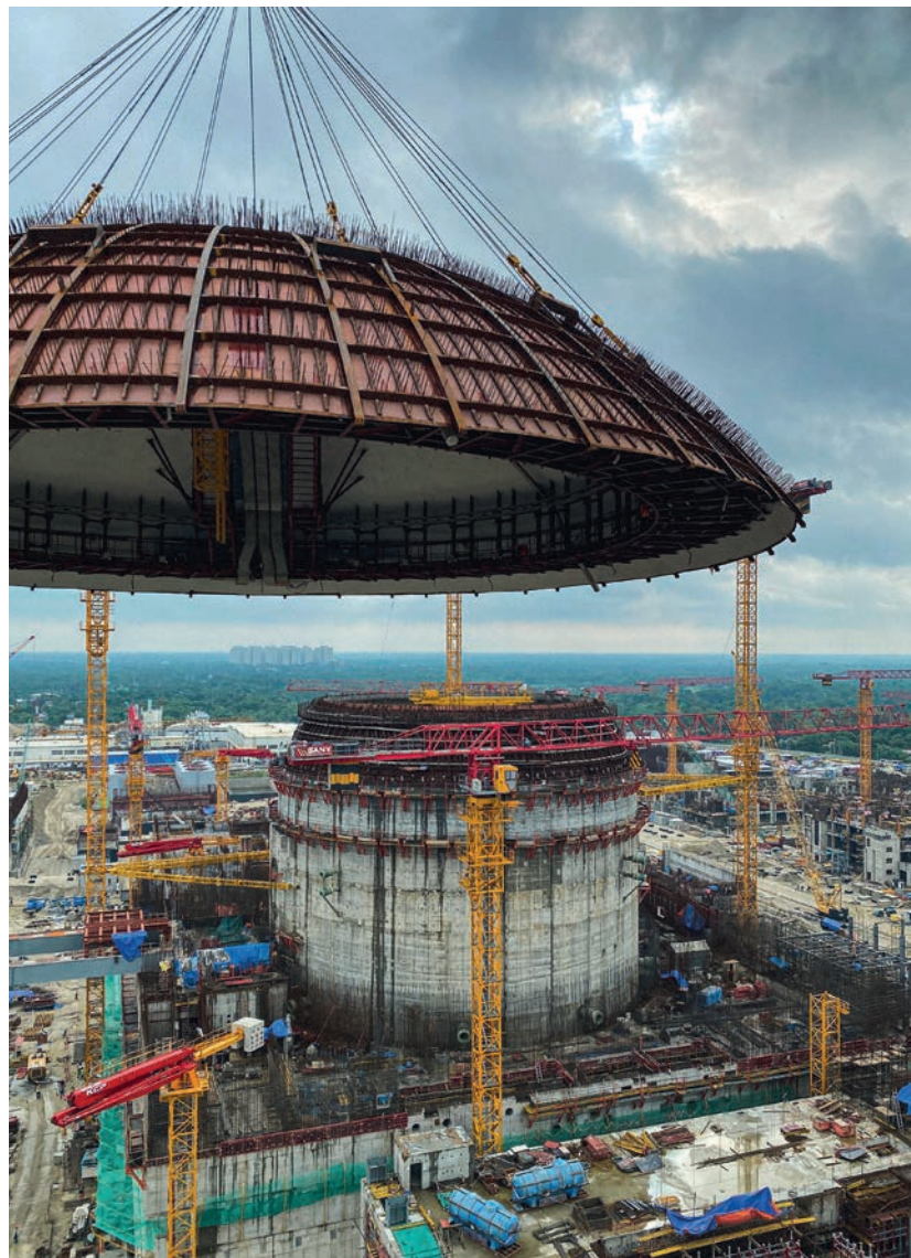
Rooppur under construction (Image: Trest RosSEM)
