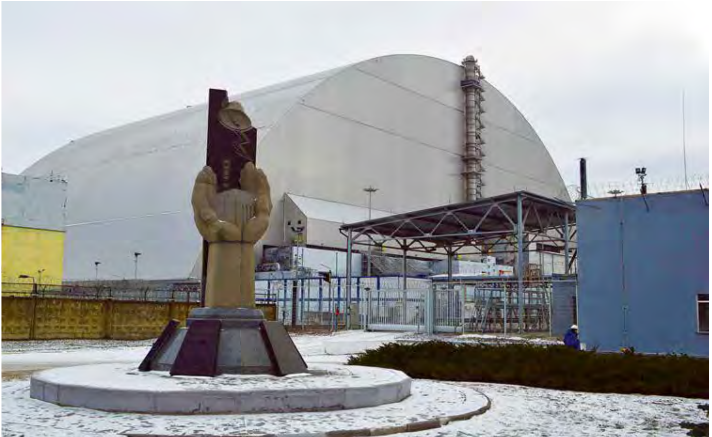
The 1986 explosion of the reactor containment building at the Chernobyl nuclear station in the Ukraine (then a part of the Soviet Union) was by a wide margin the worst nuclear accident in history. Pictured here is the New Safe Confinement structure built in 2017 to encase the reactor ruins and temporary shelter built in 1986 to prevent further radioactive contamination.
