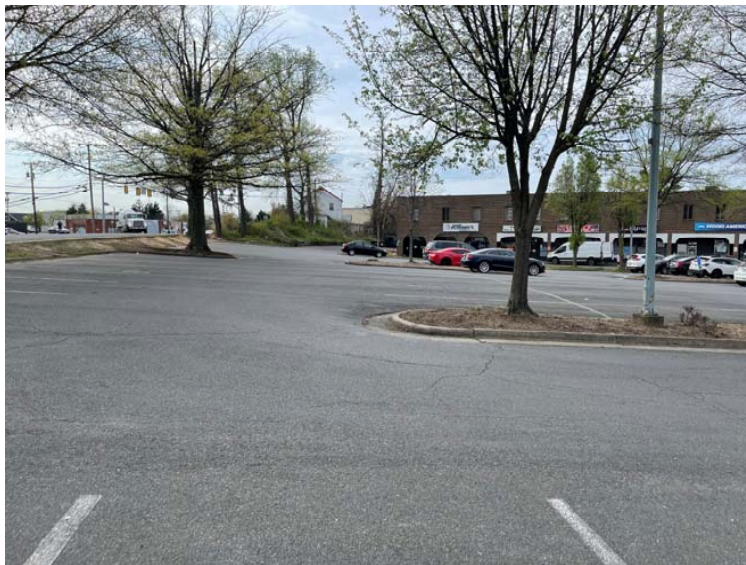
Looking toward South at the North front corner of the building, standing on sidewalk along Markham Street
