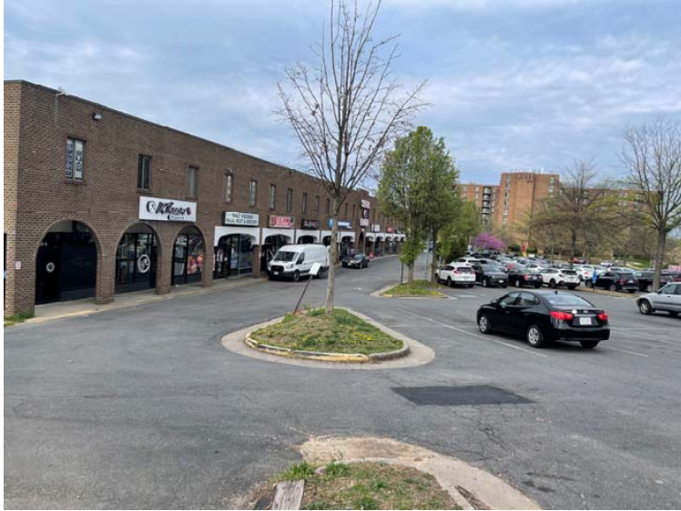
Looking toward West, at the Northeast front of the building, standing on Sidewalk along Markham Street
