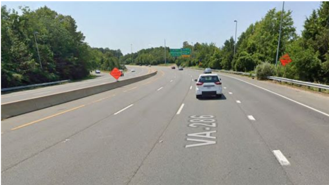
Figure 7: Fairfax County Parkway, at I-66
