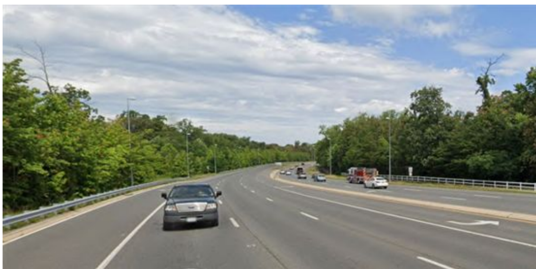
Figure 6: Fairfax County Parkway, north of Rugby Road
