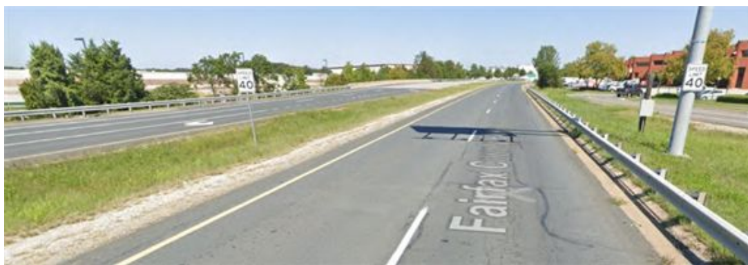
Figure 11: Fairfax County Parkway, south of I-95
