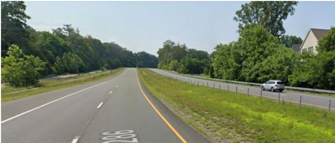
Figure 3: Fairfax County Parkway, south of Wiehle Avenue
