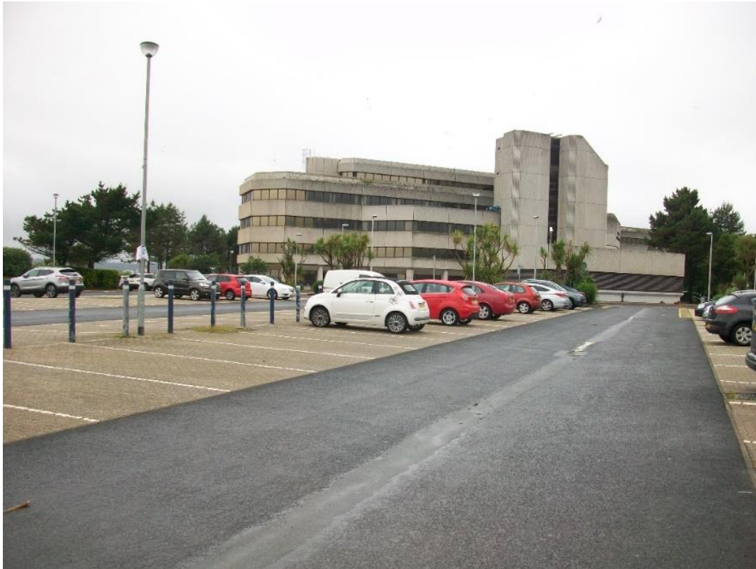
Fig 22 West Glamorgan County Hall, Swansea
