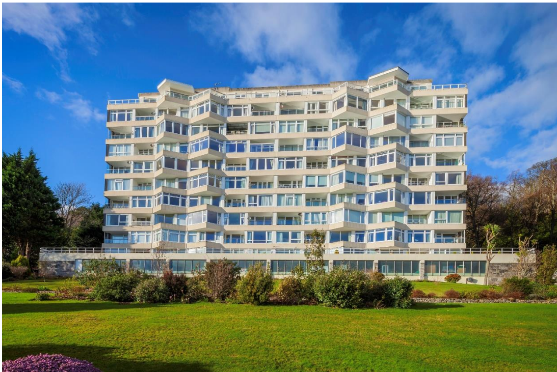
Fig 5 Glyn Garth Court, Menai Bridge © Crown Copyright (2019) Cadw Welsh Government
