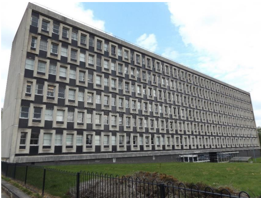
Fig 20 Flintshire County Council offices, Mold
